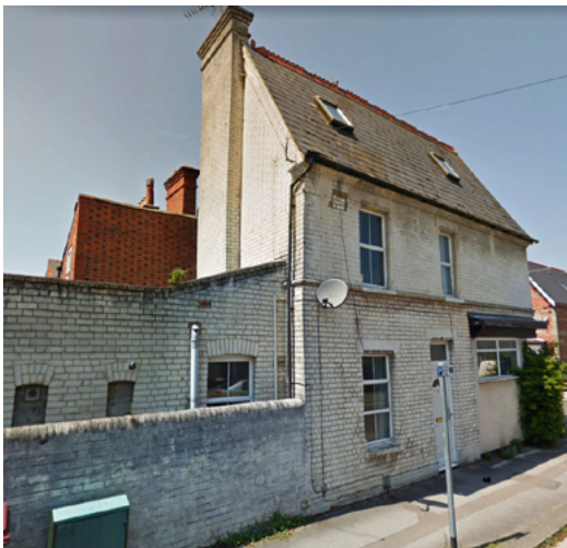
Fig.15: 30 Highgrove Street prior to refurbishment - view from the east
