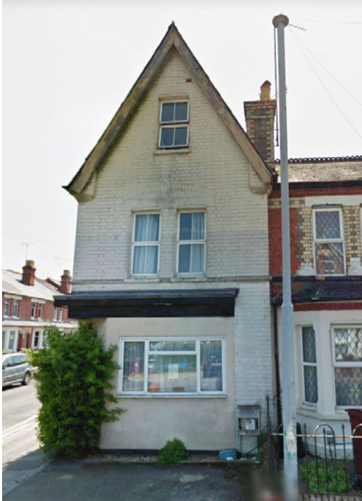
Fig.13: 30 Highgrove Street prior to refurbishment - view from the north
