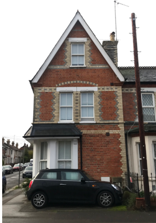
Fig.14: 30 Highgrove Street after refurbishment - view from the north
