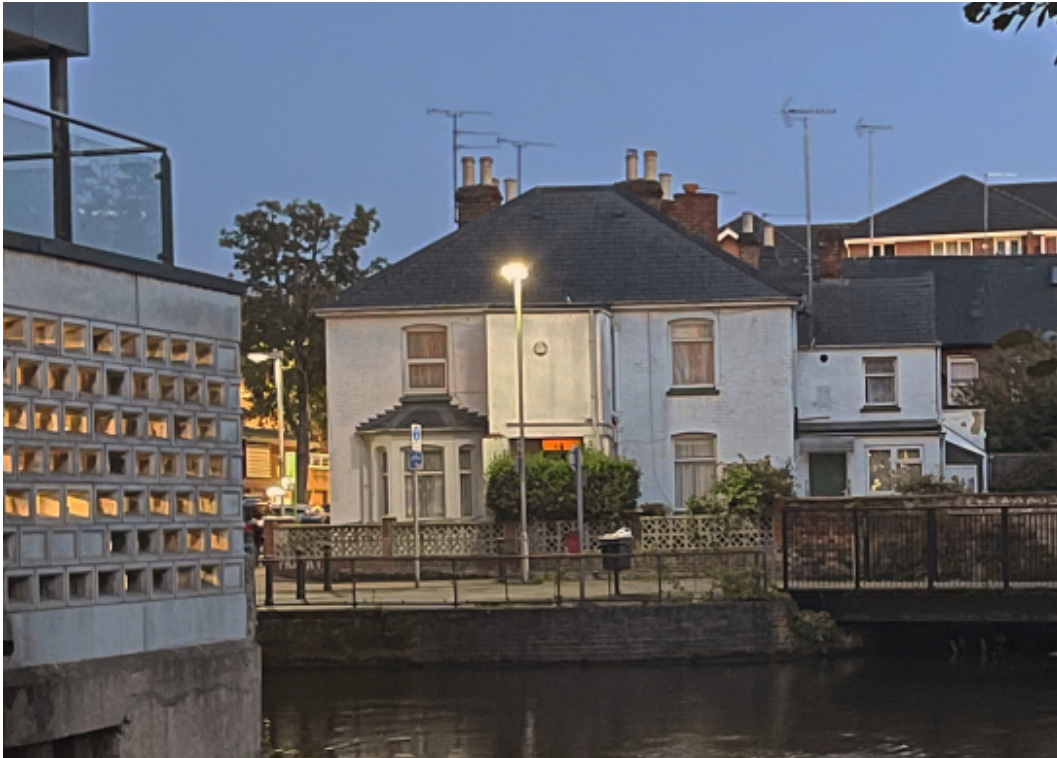
Fig.1: Existing view of 2 Sidmouth Street from across the River Kennet
