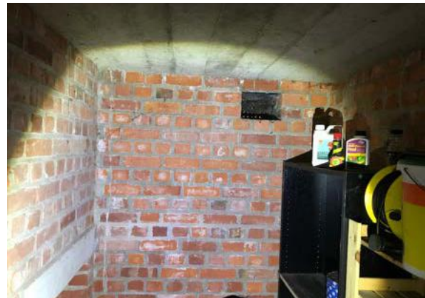
Image 8: Interior of air-raid shelter building
