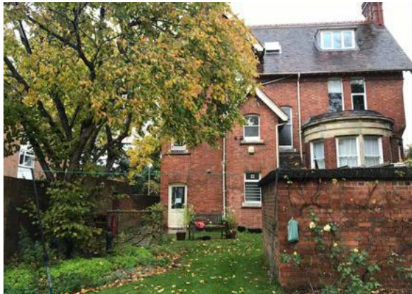
Image 1: Main building, with hazel tree and air-raid shelters to be removed
