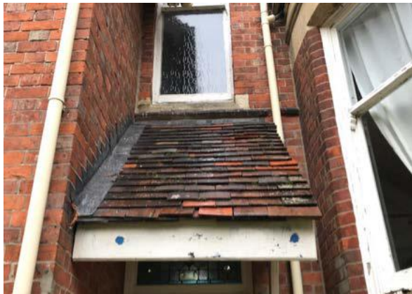
Image 7: Clay tiled porch roof
