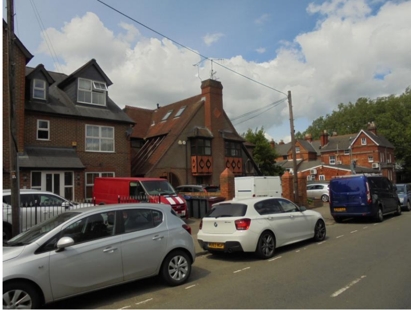
Photo 2, Photo of front elevation
