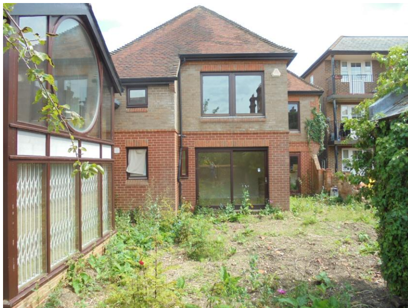
Photo 4 Photo of rear elevation
