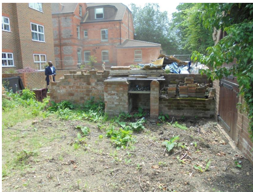
Photo 5 Rear wall to be removed
