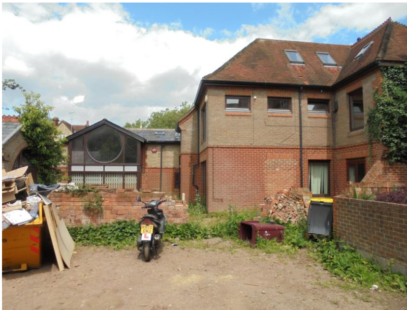
Photo 3 Side elevation addressing car park.
