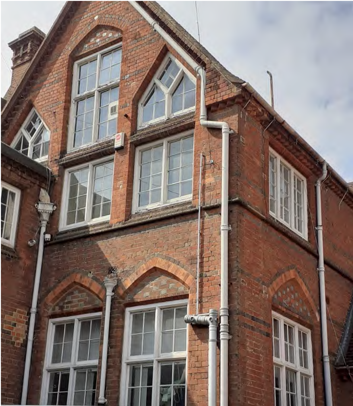
2.4.6 - .9 East Elevation 1 / North Elevation 2 Brickwork
