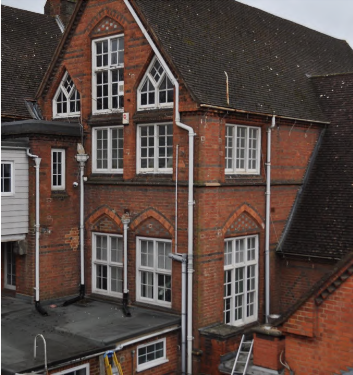
2.5.5 - .10 Elevation 1 / North Elevation 2 Downpipes
