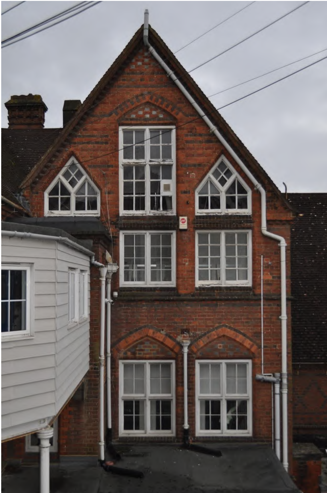
2.2.9 - .33, 2.2.55 - .59 East Elevation 1 Central Gable windows
