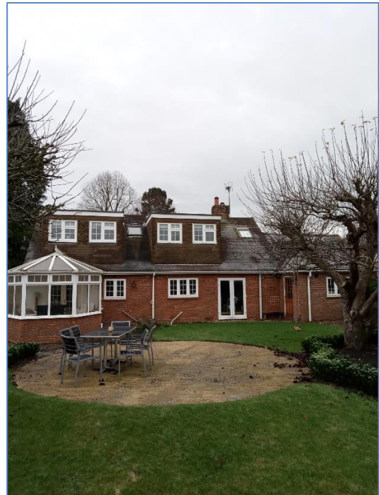
Fig 2. Existing rear elevation. Site photo taken on 06/01/2022.
