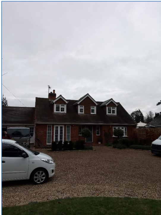
Fig 1. Existing front elevation. Site photo taken on 06/01/2022.
