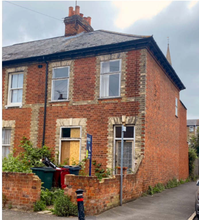
Fig 1. View from the front of the existing house.
