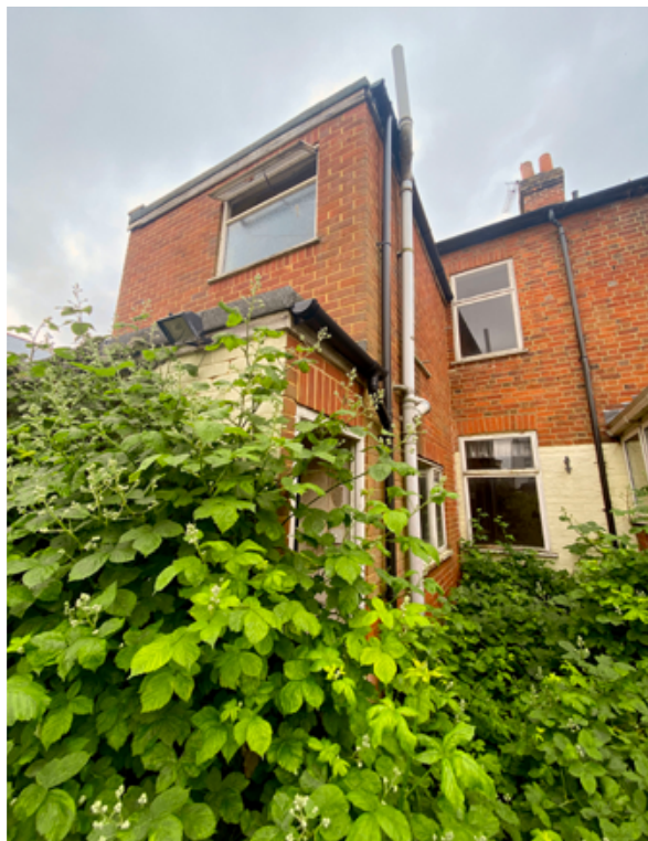
Fig 6. View of the rear of the building
