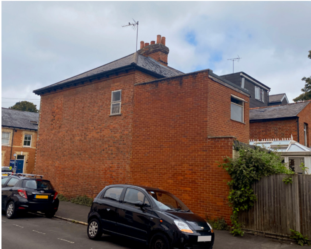
Fig 13. View of the south elevation showing existing 2 storey extension
