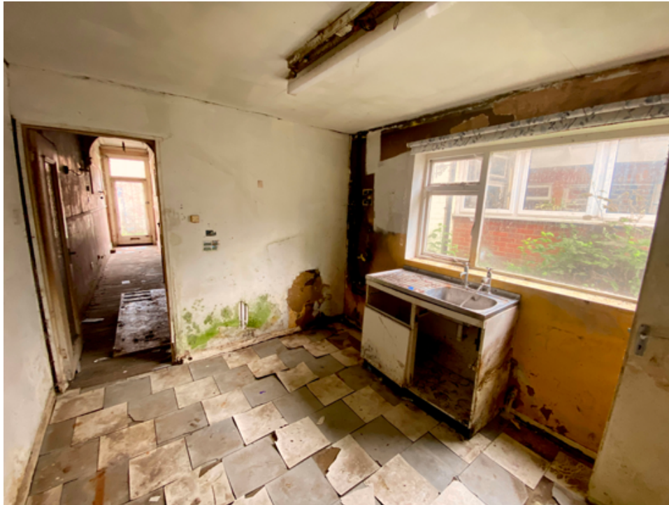
Fig 7. View of existing kitchen area
