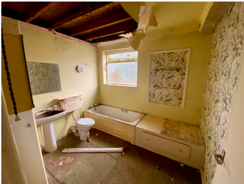
Fig 8. View of existing bathroom
