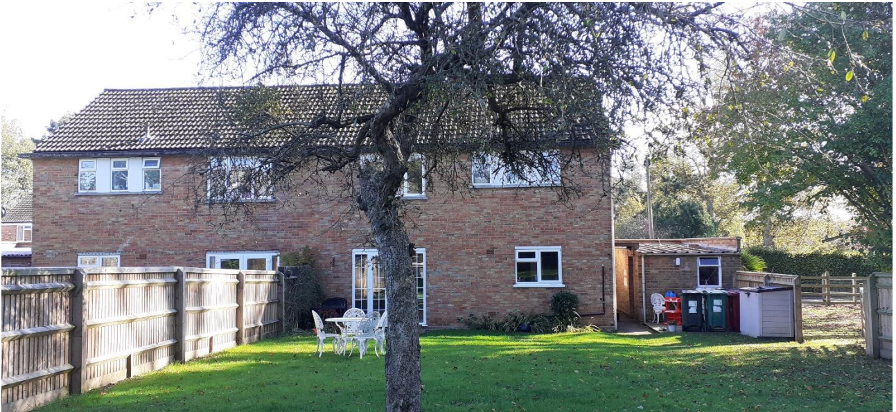
REAR OF 25 HEWETT AVENUE
