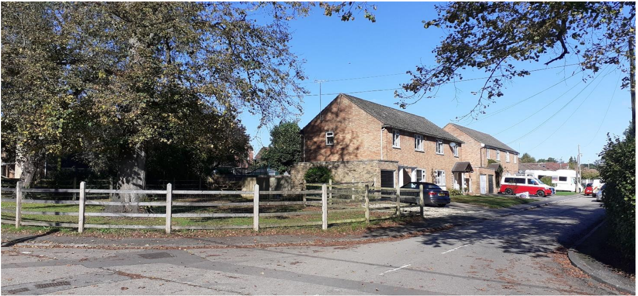
LOOKING NORTH TOWARDS SITE FROM CHAZEY ROAD
