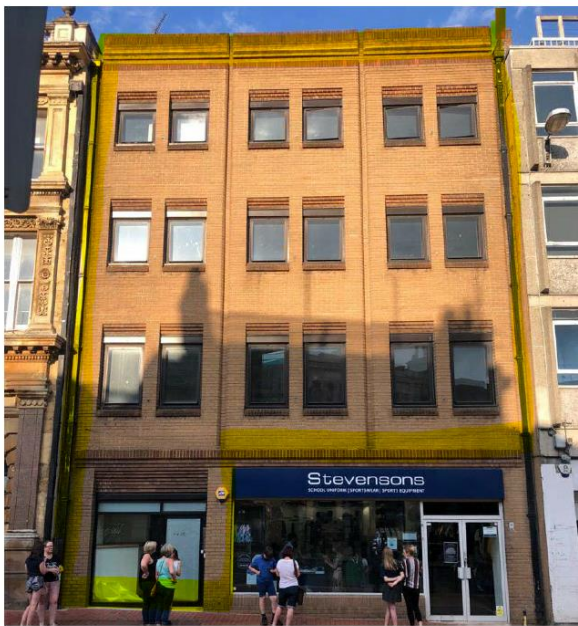
Photograph of the existing front of 11 - 12 Market Place.
