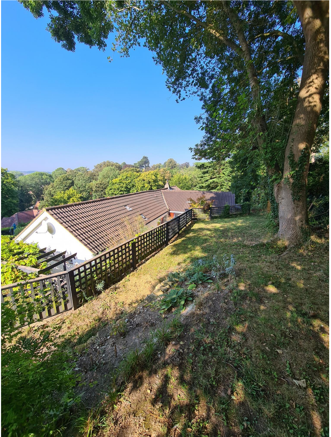
View from raised part of the garden looking toward the proposed south-east facing window to serve an ensuite.
