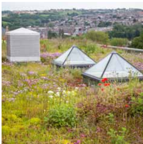
Figure L46: Biodiverse green roof
