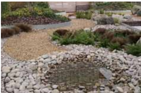
Figure L47: Biodiverse green roof Example of a biodiverse roof with a variety of substrates and standing water.
