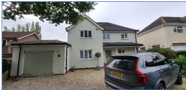
1. Front of 31 Chazey Road. Photo provided by agent on 17/12/2020.
