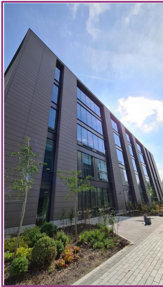
Figure 3: Existing Northern Office Block
