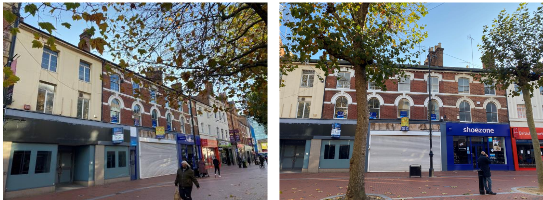
Figures 24 and 25: Broad Street elevations of nos. 86-87
