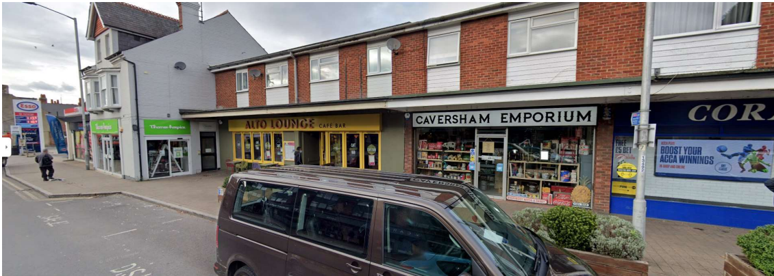
View along Church Street illustrating its commercial nature at ground floor
