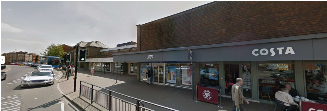
View along Church Street illustrating its commercial nature at ground floor
