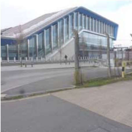
2. Railway station, northern entrance
