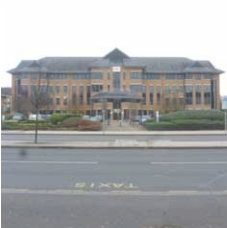
2. Office Building on Vastern Road
