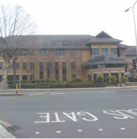
3. Office Building on Vastern Road
