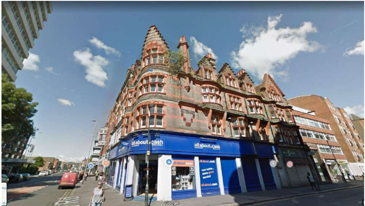
Figure 2 Source: Google Street View
