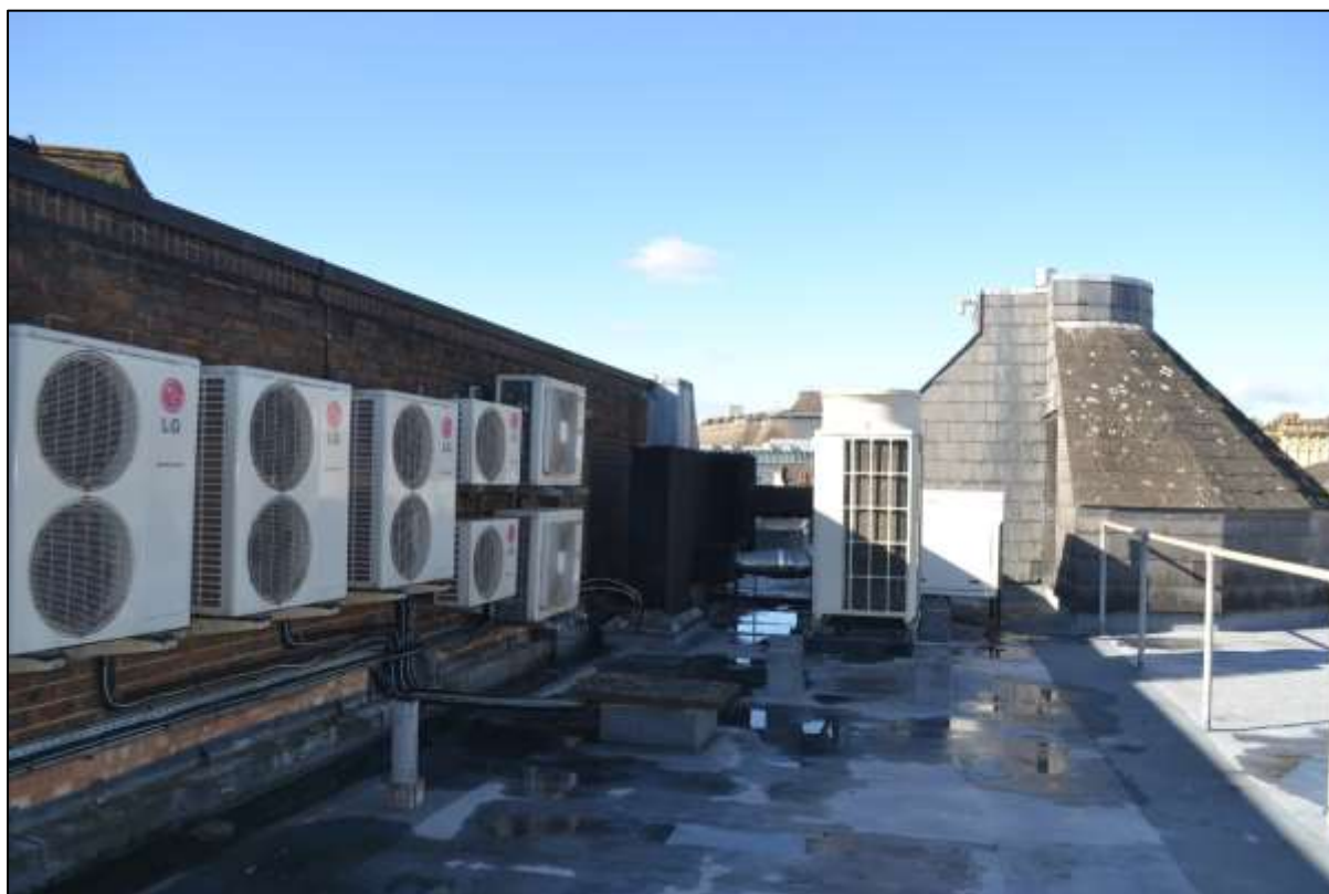
Figure 25: Photograph of the existing roof and plant room
