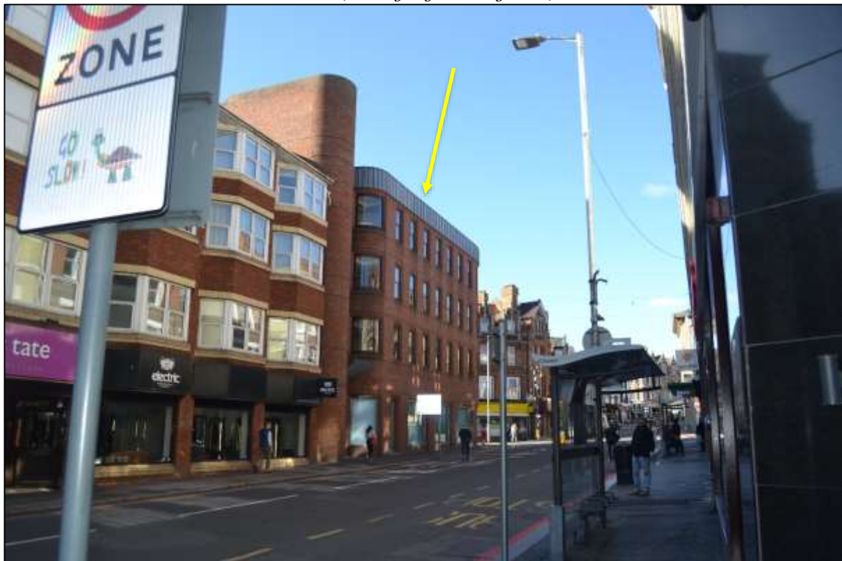
Figure 22: View of 2-4 Kings Road looking west along Kings Road (site highlighted in yellow)
