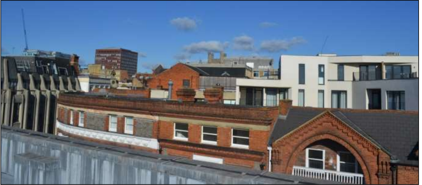
Figure 41: Various roof extensions and rooflines when looking north from the roof of 2-4 Kings Road
