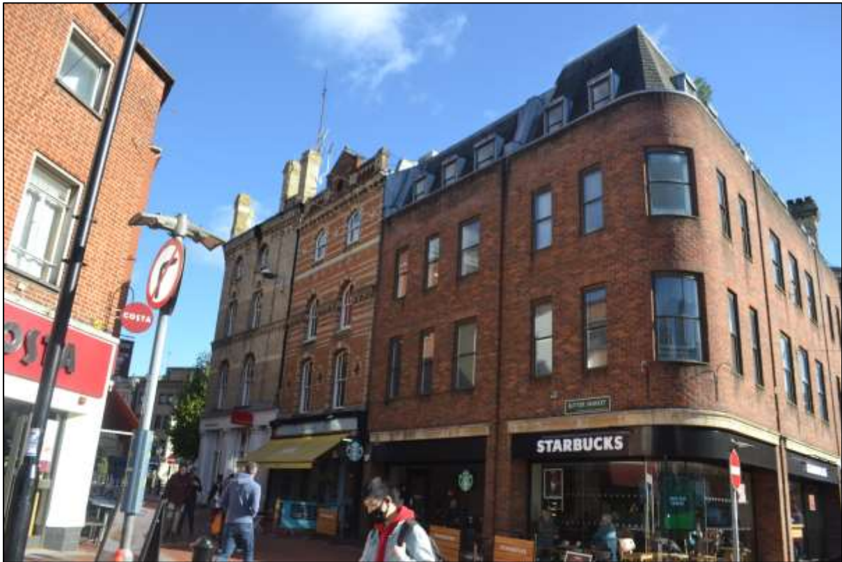
Figure 37: Roof extension to building located to the west of the site along King Street
