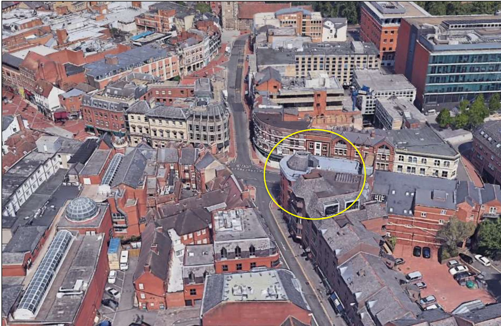
Figure 6: Aerial view of 2-4 Kings Road highlighted in yellow looking north
