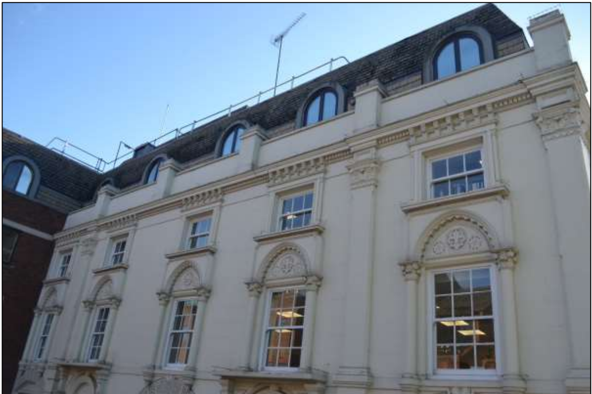
Figure 40: Roof extension to Grade II listed Coroners Corner south of the site along London Street
