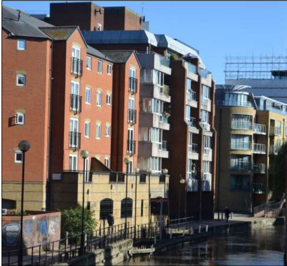
Figure 35: Further examples of roof extensions to buildings along the river front to the south of the site
