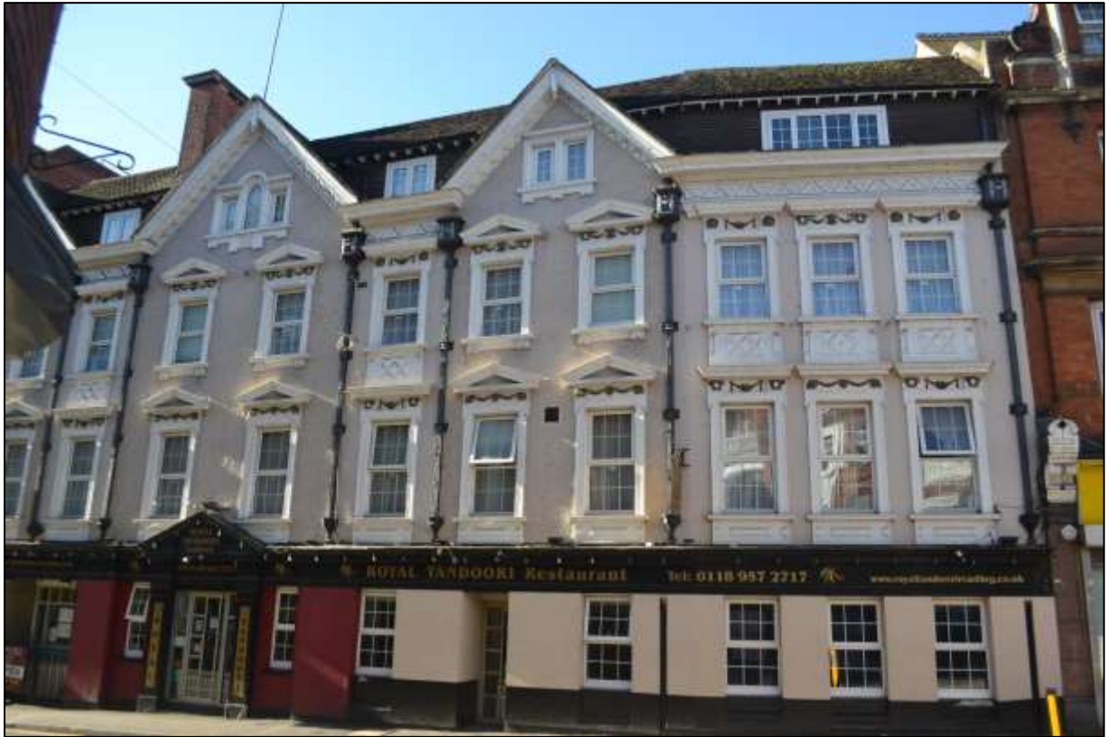
Figure 33: Roof extension to building of townscape merit opposite the site to the west
