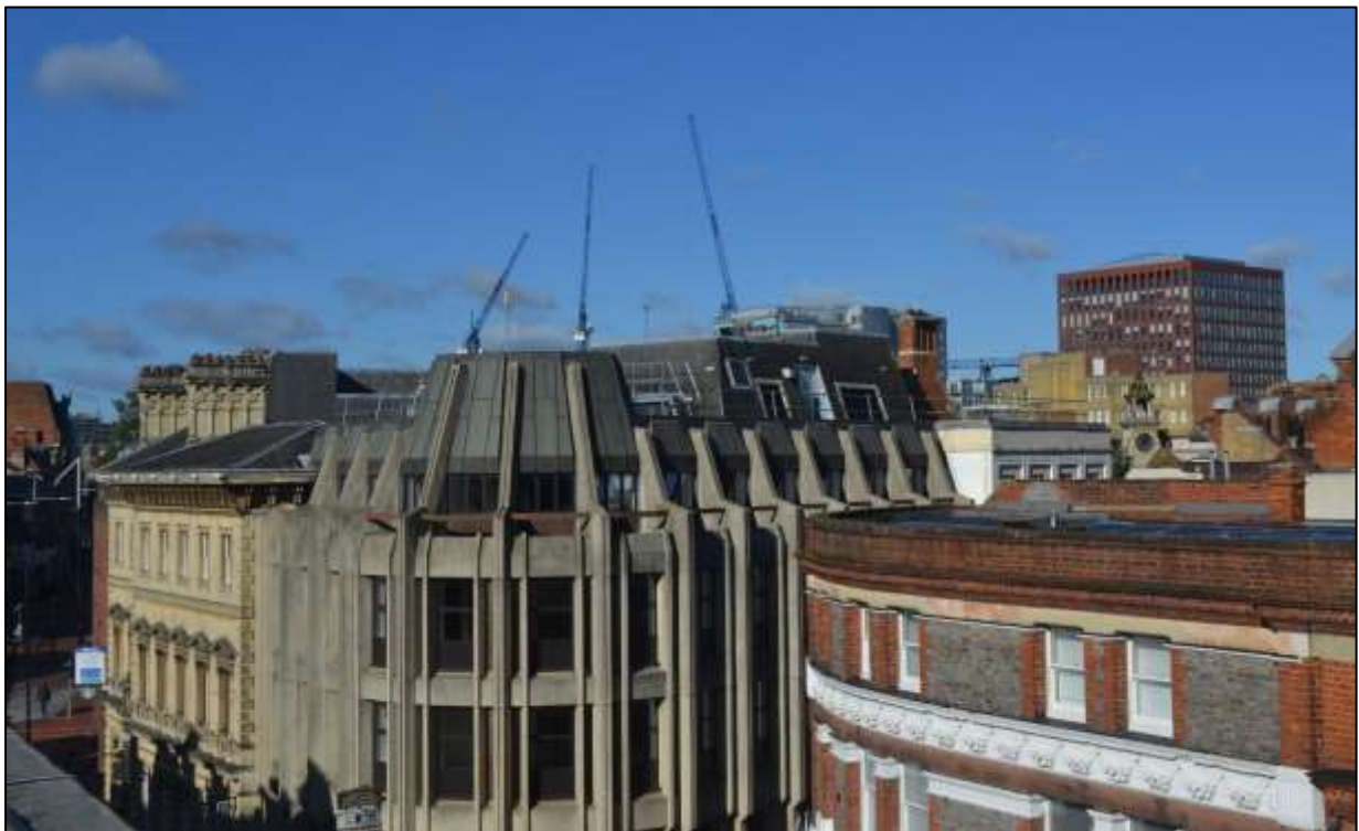
Figure 34: Roof extension to building opposite the site (north-west)- seen from roof of 2-4 Kings Road
