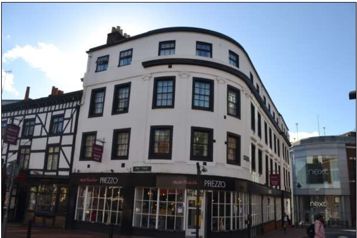
Figure 38: Roof extension to Grade II listed George Hotel to the west of the site along King Street
