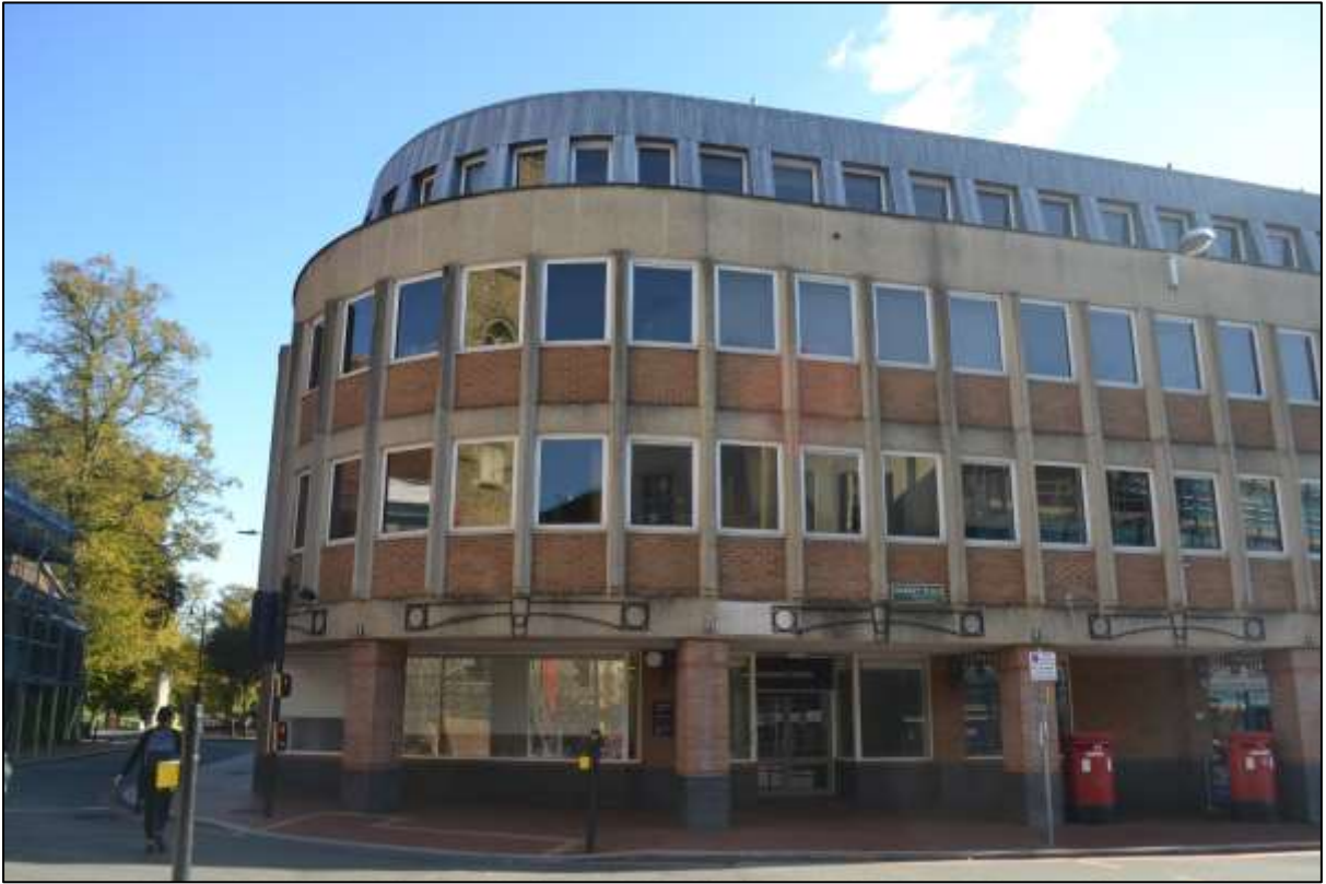
Figure 39: Roof extension to building north west of the site along Market Place
