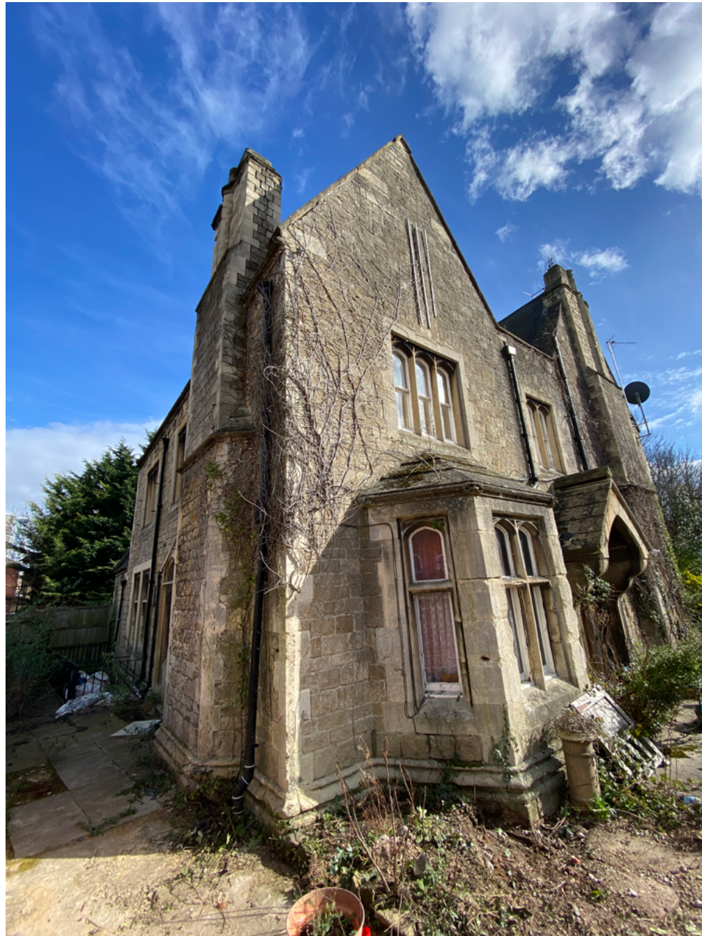
Fig.32: View of Carlisle House with gothic details from the north west
