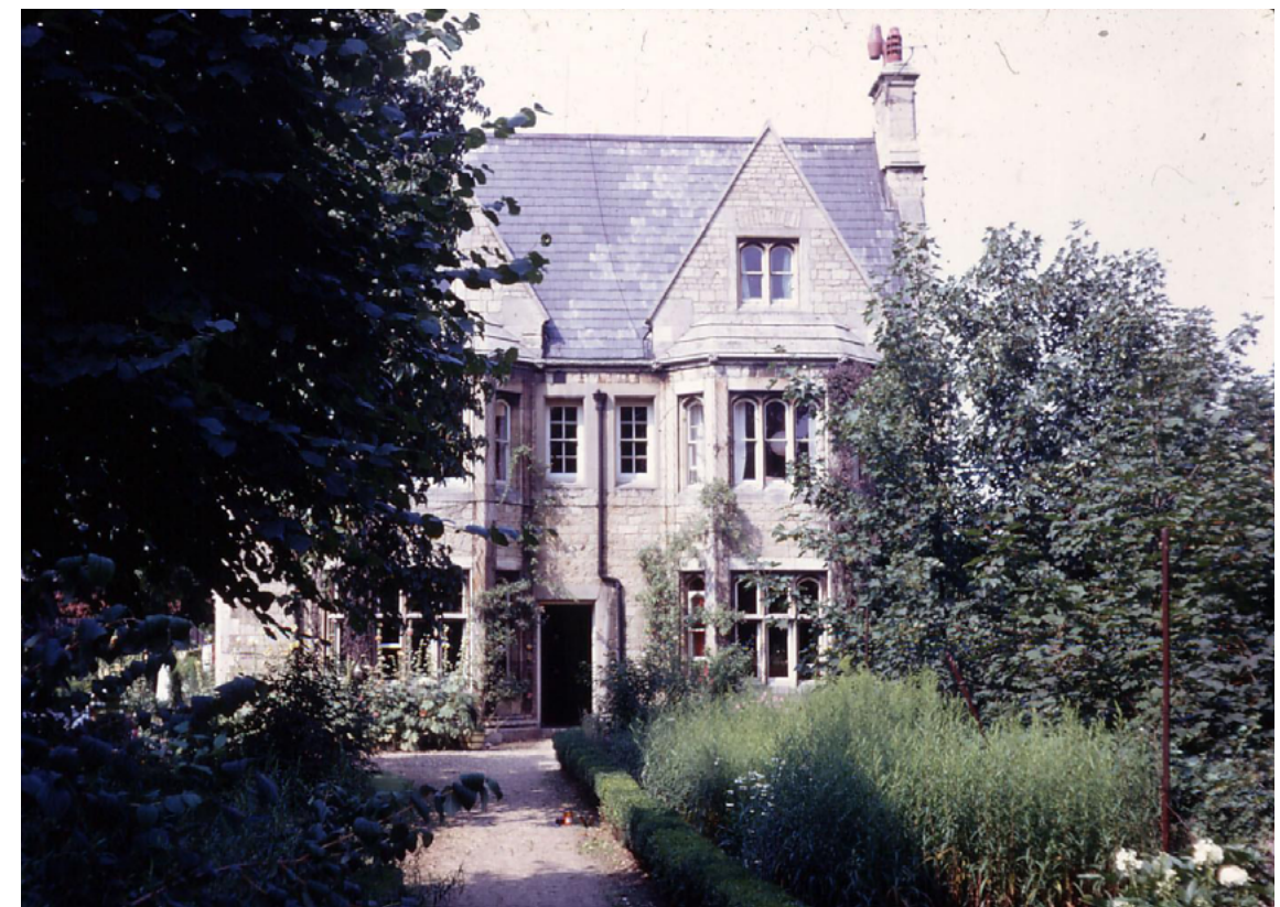
Fig.33: View of Carlisle House south elevation from 1970, following flat conversion but prior to removal of chimney stacks.
