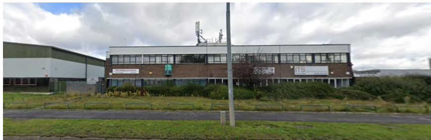
View of site frontage
