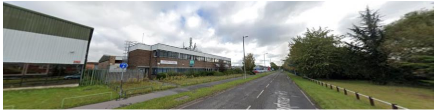
Looking east towards the site
