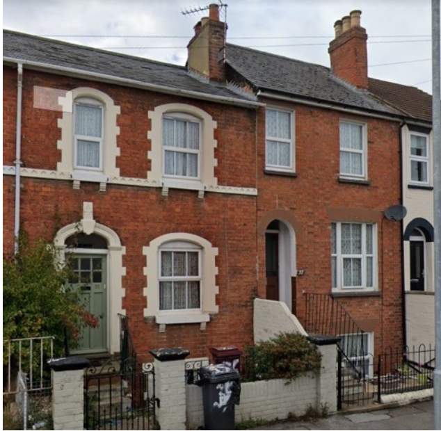
1. Front elevations of 35 and 37 Bedford Road houses.
