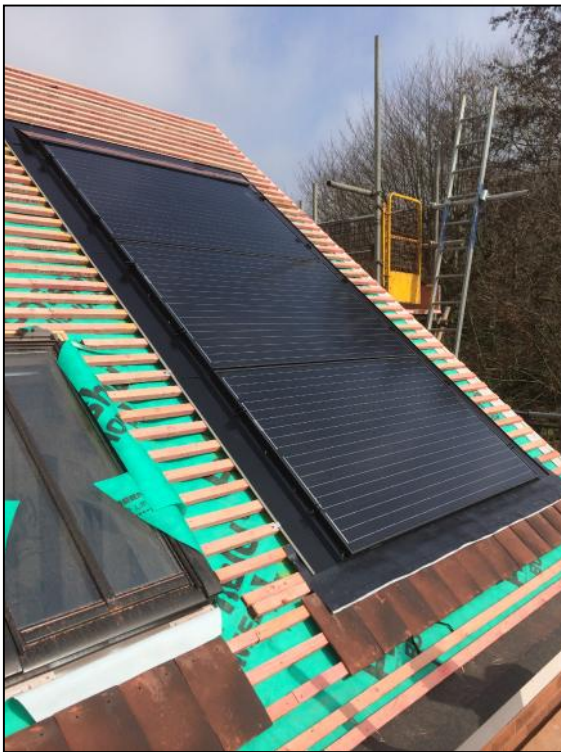
Photovoltaic Panels (in roof system)
