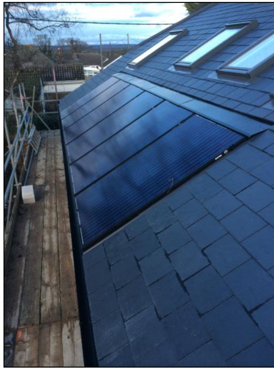
Photovoltaic Panels (in roof system)
