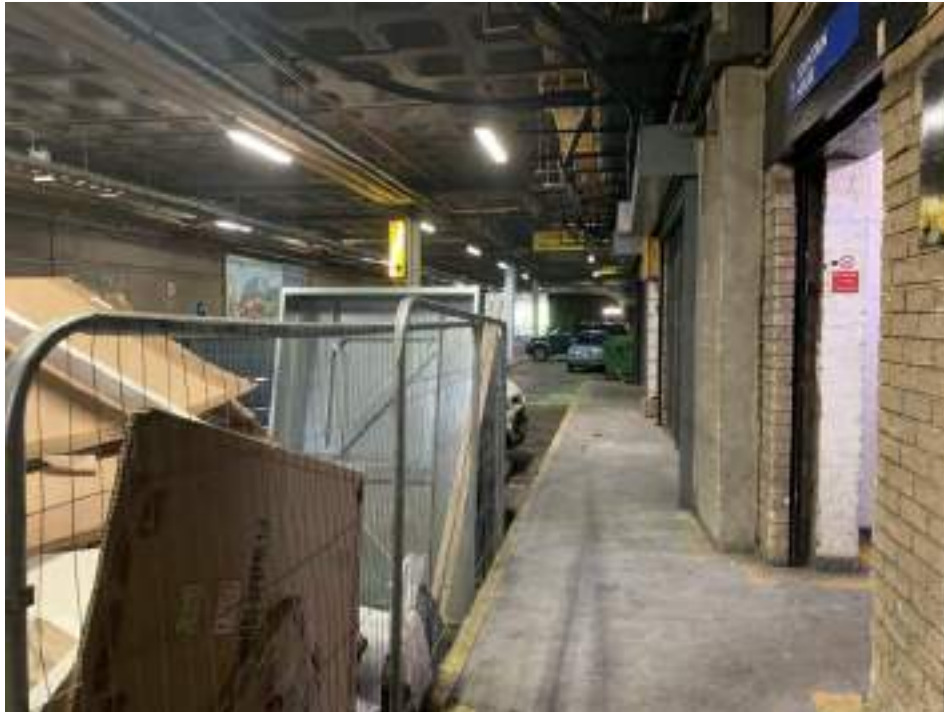
Photo 3: Entrance to Fountain House from the basement shared with the Broad Street Mall.
