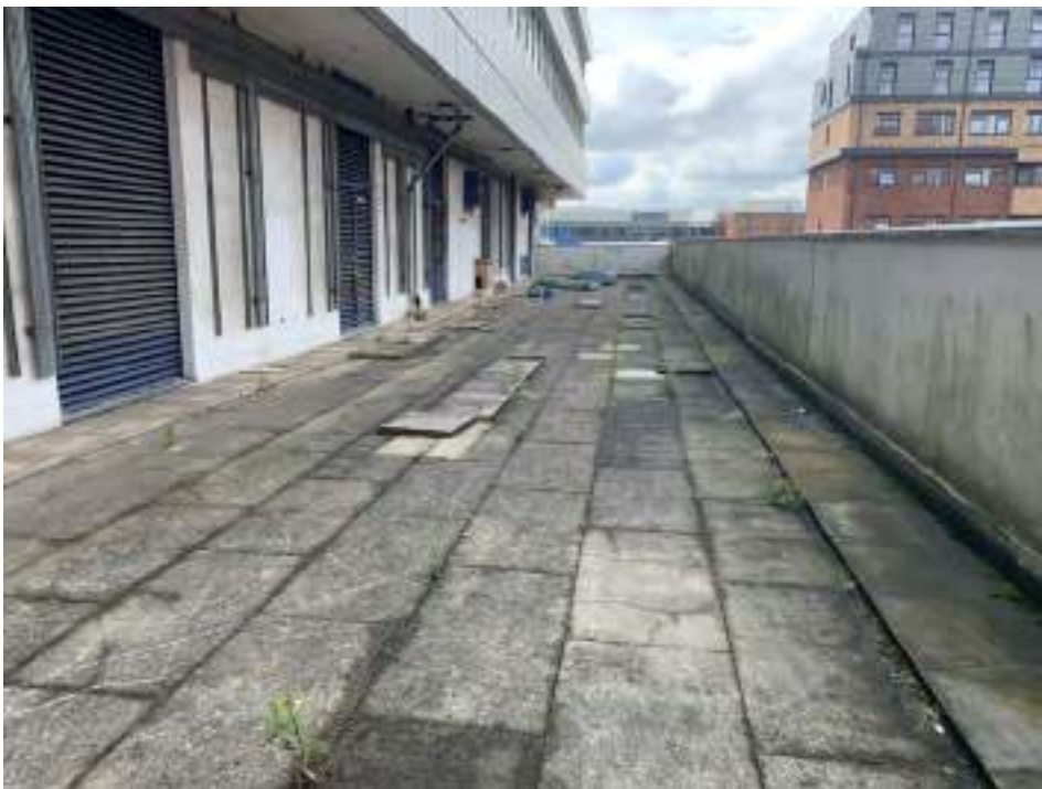
Photo 4: Off-site external area that provides access to the plant rooms on Level 2.
