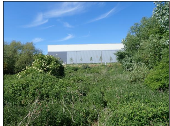
Photo 2 General view of site looking north
