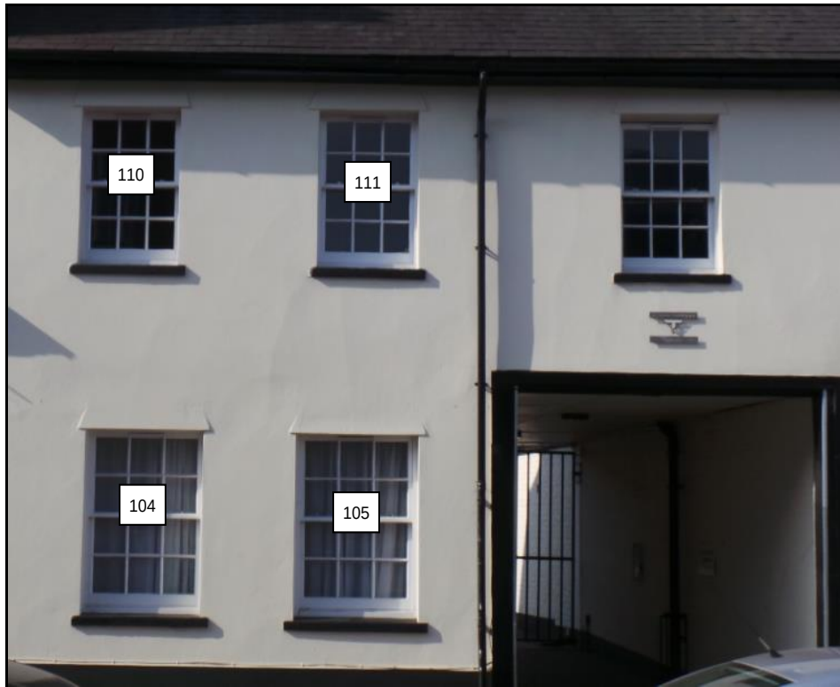
104 and 106 Southampton Street
