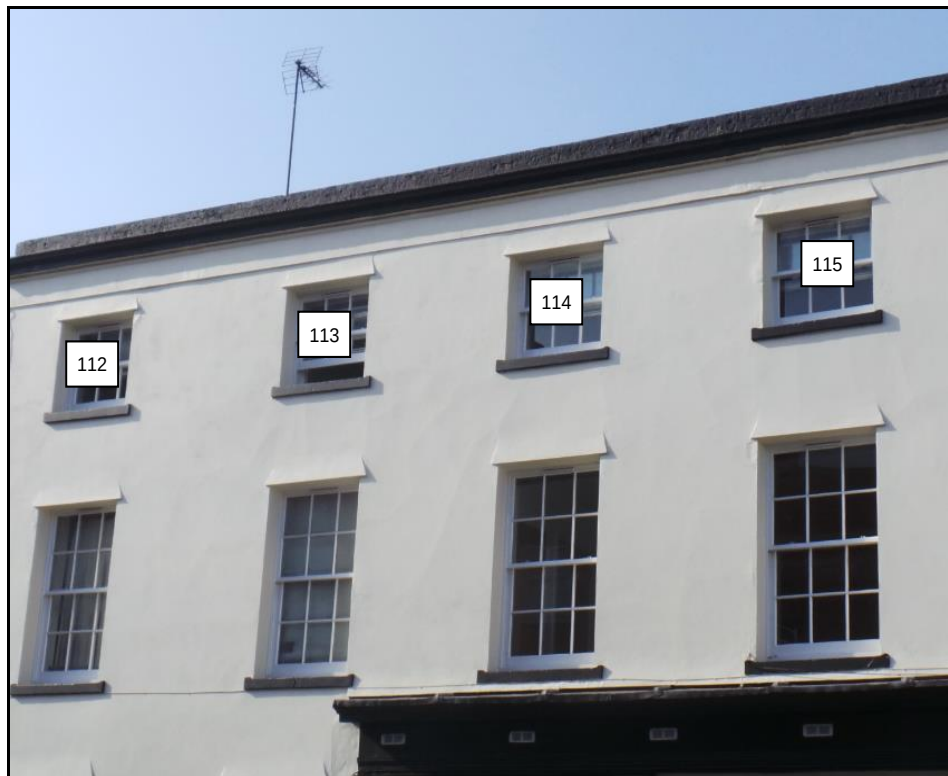
104 and 106 Southampton Street
