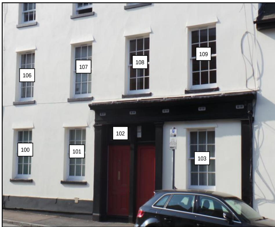
104 and 106 Southampton Street
