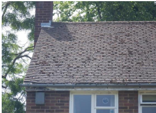
6. Ridge tiles all in place and mortared.
