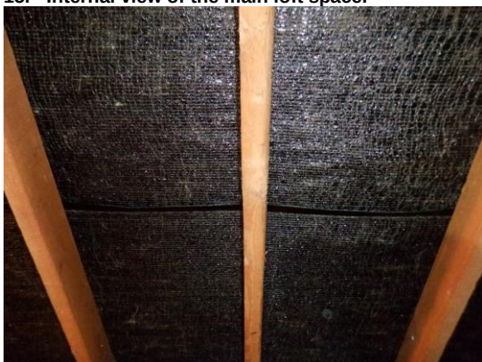
17. Roof tightly lined with bitumen felt.
