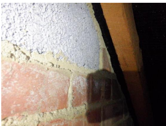
23. The side gable ends of block work and brick work construction, with cement filling the gaps around the edges.
