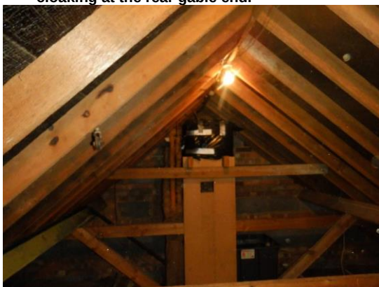
15. Internal view of the main loft space.
