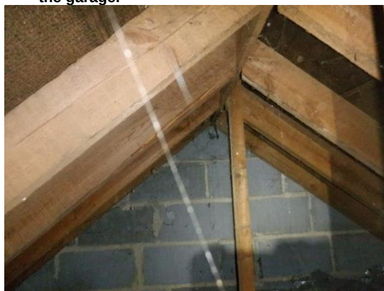
16. Internal view of the rear gable end.
