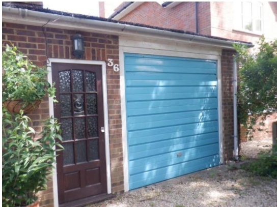
3. Flat roof garage attached to the eastern side of the house.
