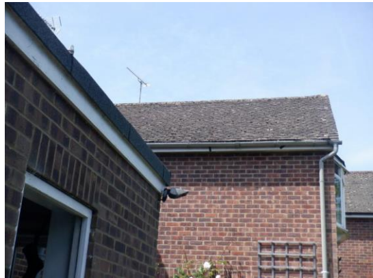
4. Roof tiles mostly tight to the rear of the house.
