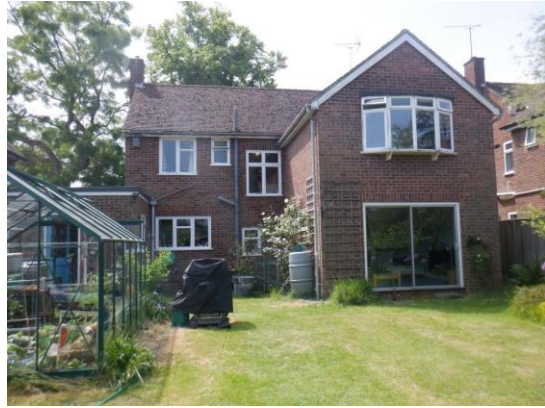
2. Rear of the house viewed from the north.
