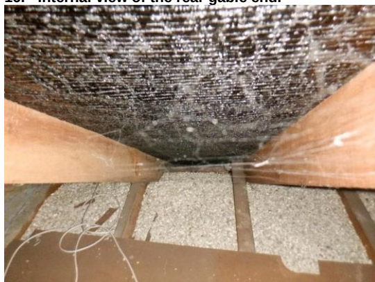
18. The floor insulated with vermiculite.
