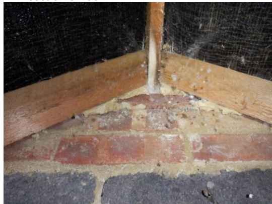
22. The side gable ends of block work and brick work construction, with cement filling the gaps around the edges.
