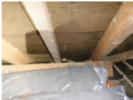
20. The eaves filled with fibreglass in the rear section of roof.
