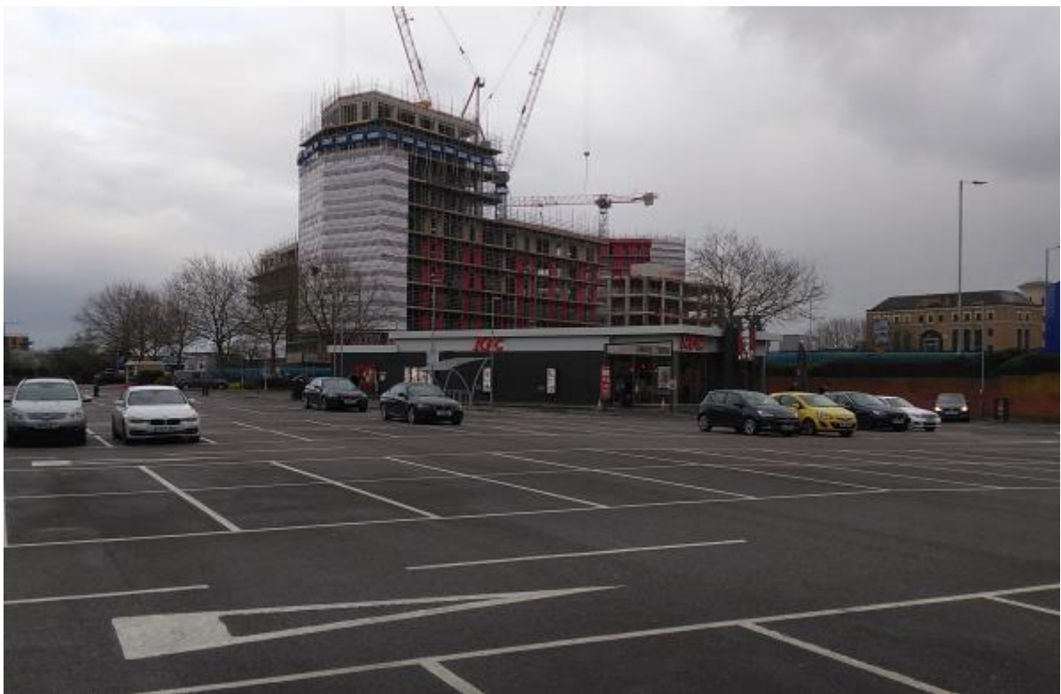
North and West elevations of the under construction Block M2 from the nearby retail park car park (photograph taken on 03/02/2021)
