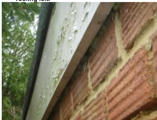
12. Gaps behind timber fascias on the eastern side of the garage.
