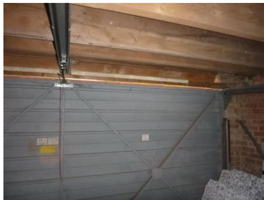
26. Gap present at the top of the garage door.
