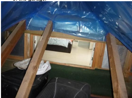
15. Internal view of eaves space 1 with a south facing gable end.
