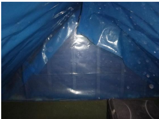
19. Hanging tiles covered with plastic at the southern gable end in eaves space 1.
