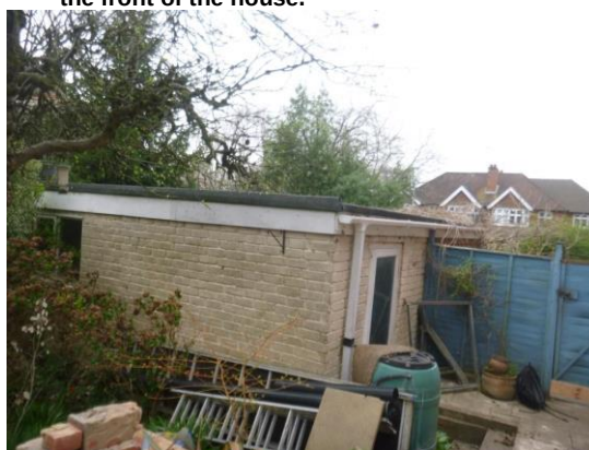
10. Flat roof garage tightly fitted with bitumen roofing felt.
