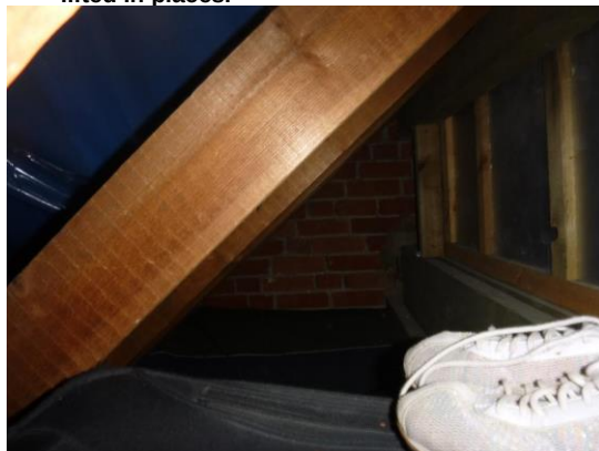
16. Brick wall at the western end of the eaves space 1.
