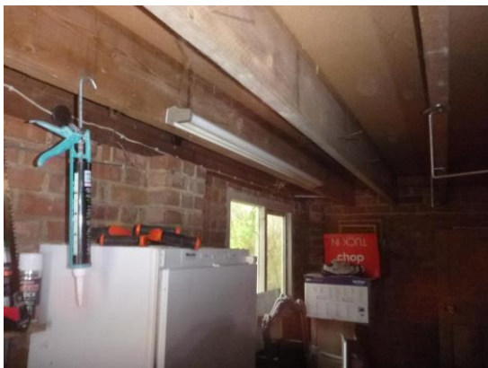
25. The internal view of the garage with hardboard tightly fitted on the roof.
