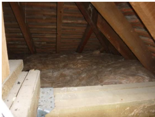
20. Internal view of eaves space 2.
