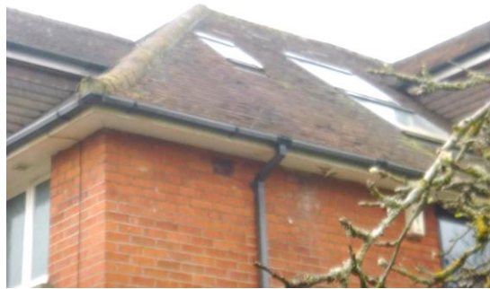
4. Roof tiles mostly fitted tightly.
