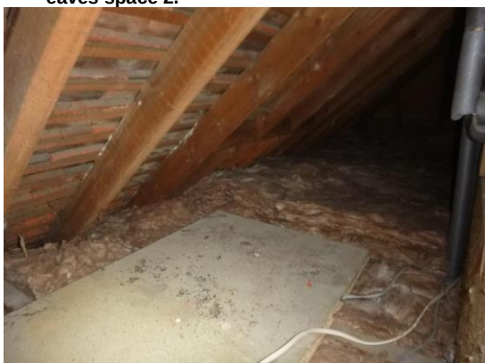
23. The boarded floor and insulation in eaves space 2.
