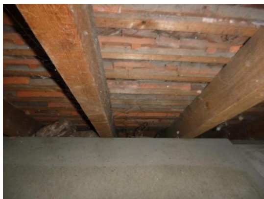
24. The open eaves in eaves space 2.
