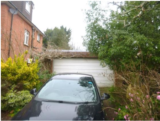
3. Detached garage to the east of the house.
