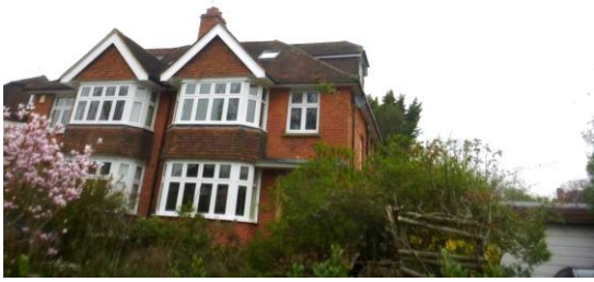
1. Front of the house viewed from the south.
