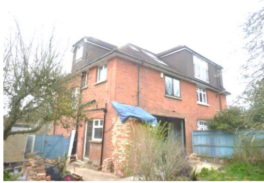
2. Rear and side of the house viewed from the northeast.
