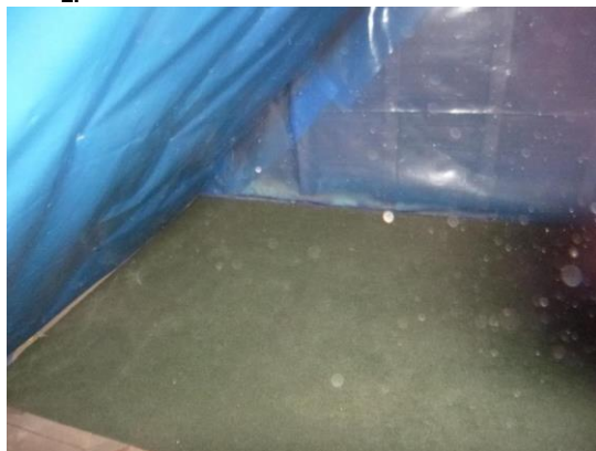
18. Floor boarded in eaves space 1.
