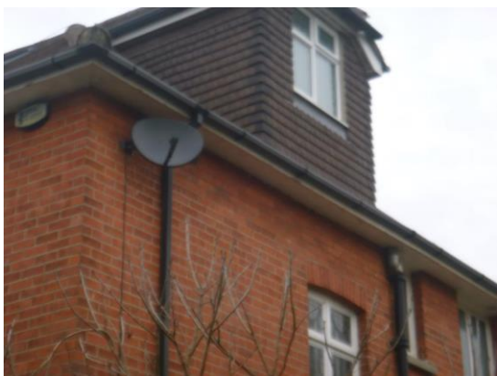
7. Timber soffits tight to the eaves.
