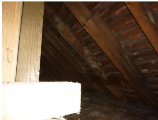
22. The unlined roof of eaves space 2.
