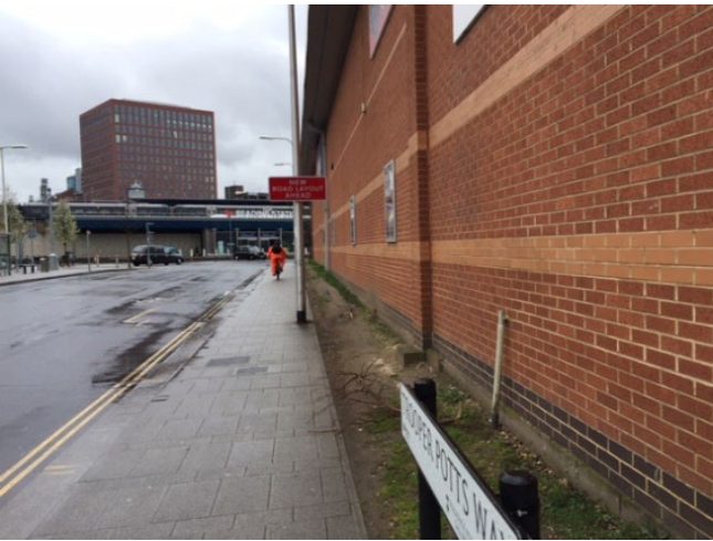
South facing view of Reading Railway Station from Trooper Potts Way
