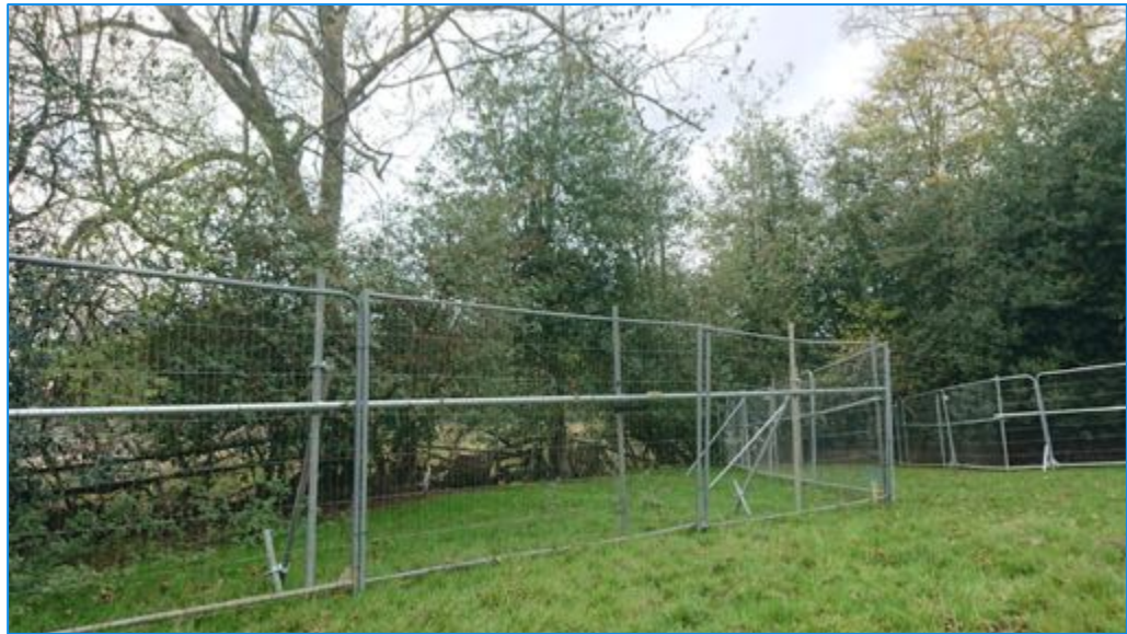
Typical tree protection barrier construction
