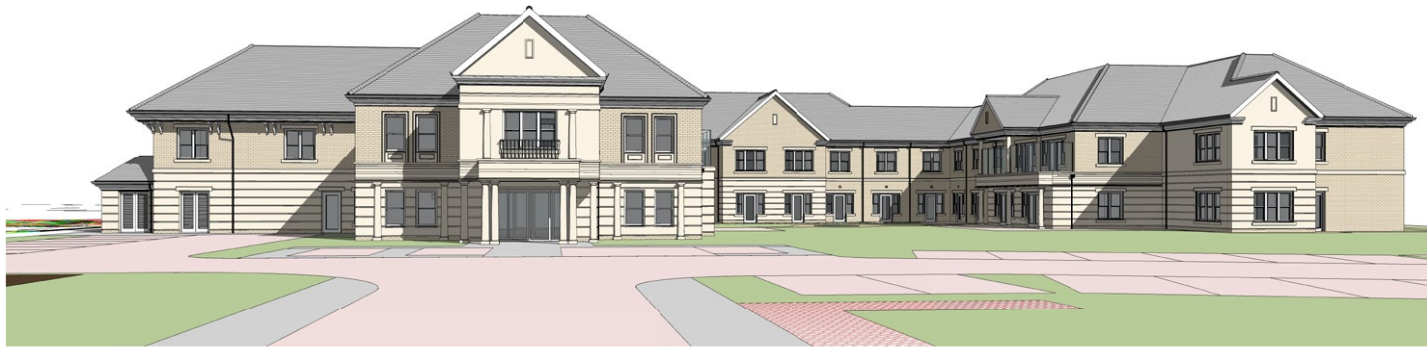
View from site entrance to the North
