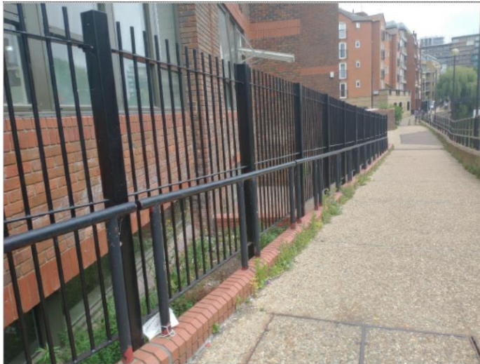
Photograph of the partly erected fence
