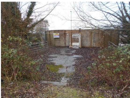
Photograph 3. View north across ditch bridge towards Smallmead Road
