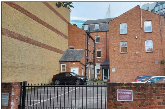
Plate 1. Rear of 58 Kings Road, looking north.
