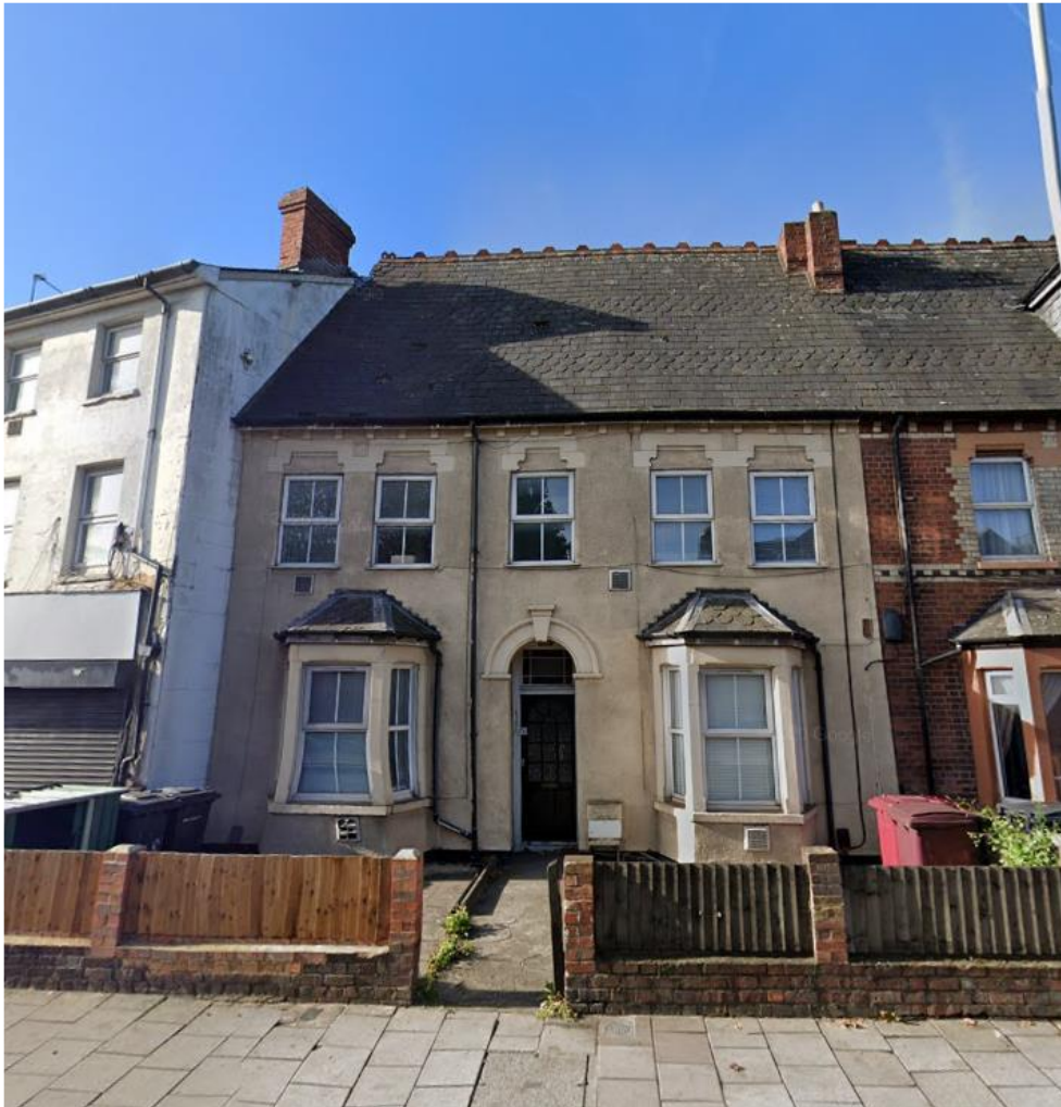
Image 9 - Street view of 119 Caversham Road
