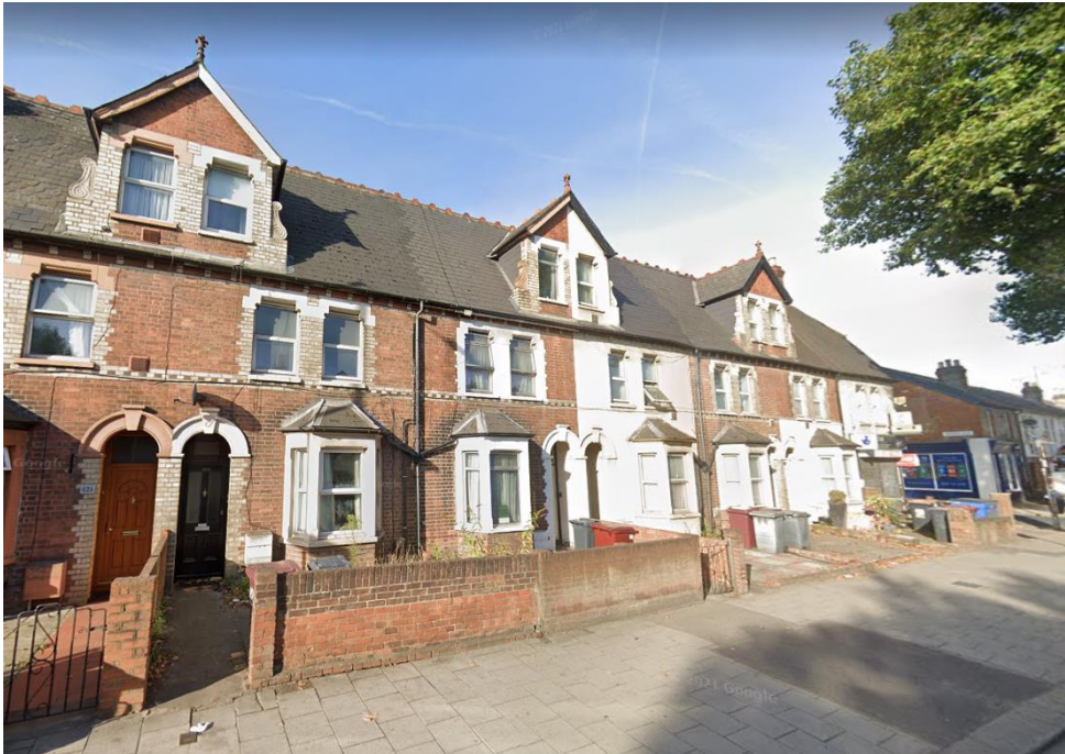
Image 6 - Street view of 123-133 Caversham Road
