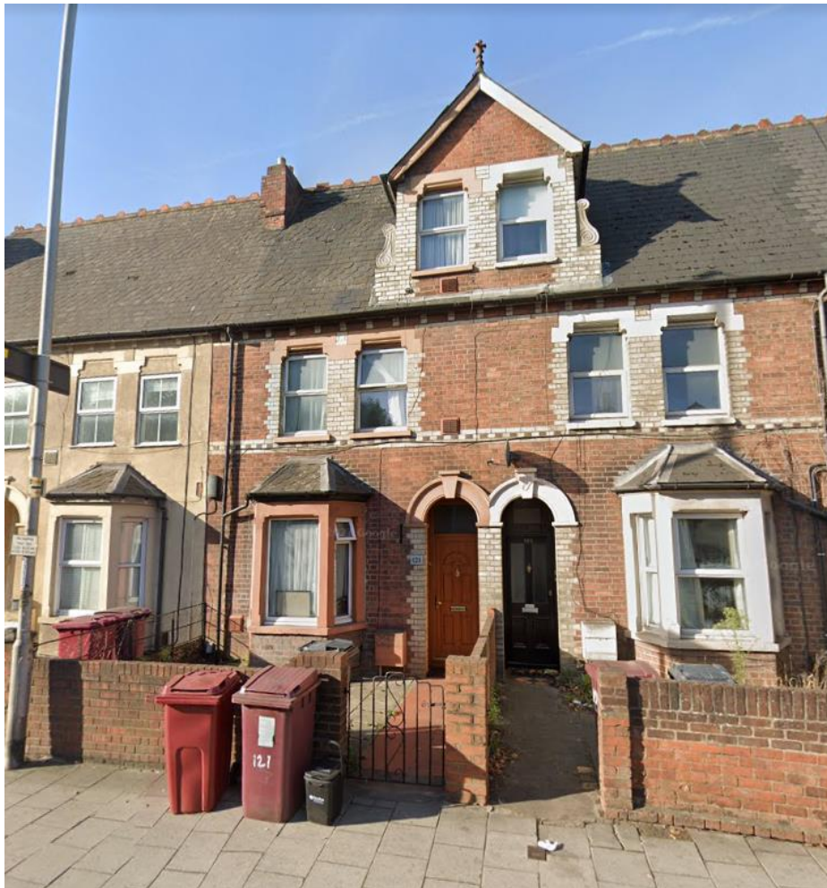
Image 7 - Street view of 121 Caversham Road
