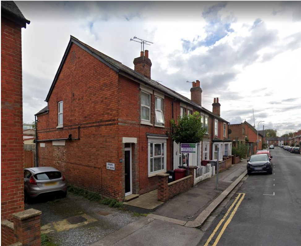
Image 4 - Street view of 32-40 Swansea Road
