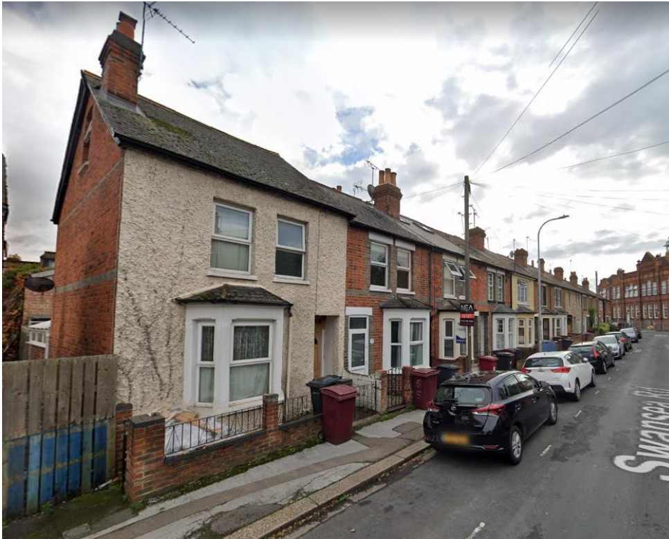
Image 5 - Street view of 42-68 Caversham Road
