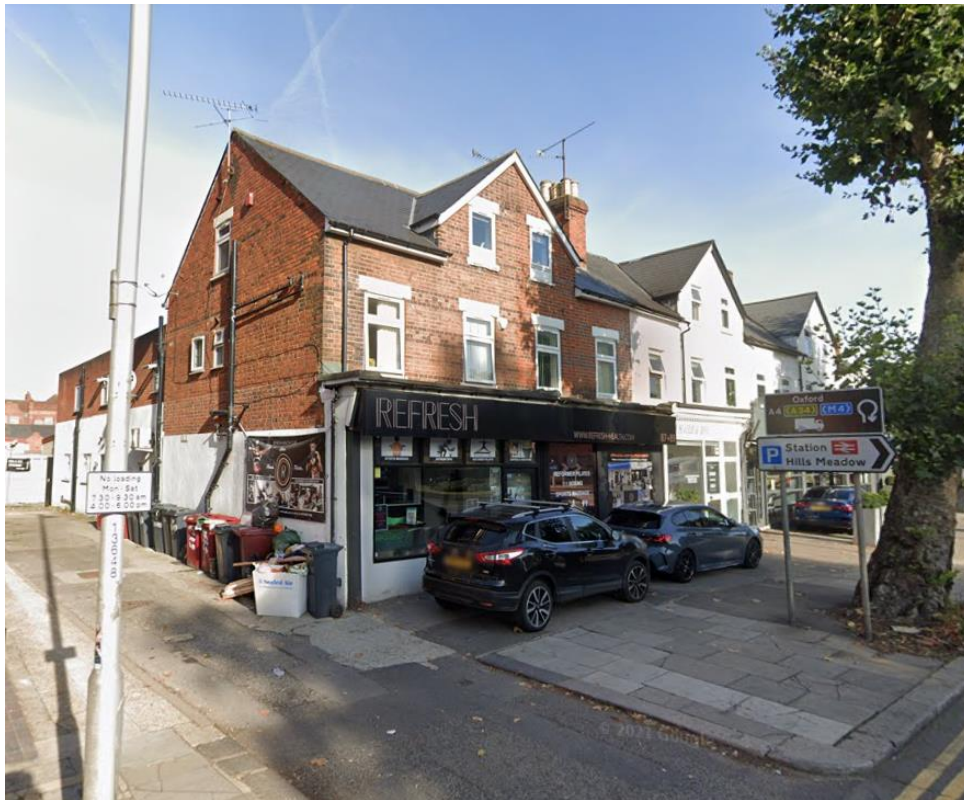
Image 13 - Street view of 87-91 Caversham Road
