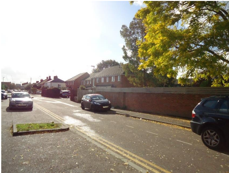
Flank wall opposite No. 68 St Johns Road
