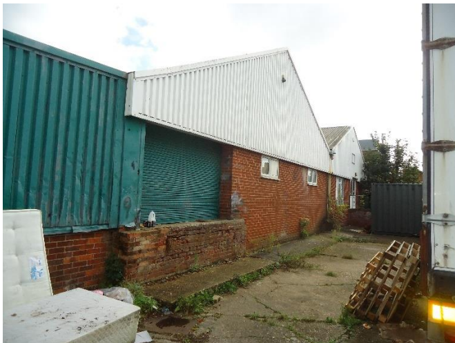
Front View of No. 68 St Johns Road (Warehouse)
