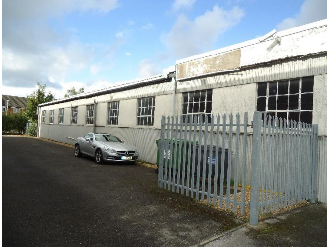
Side Perspective of No. 68 St Johns Road (Warehouse)
