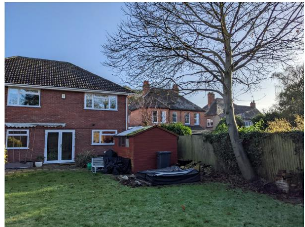
2.0 Rear elevation and tree along south boundary
