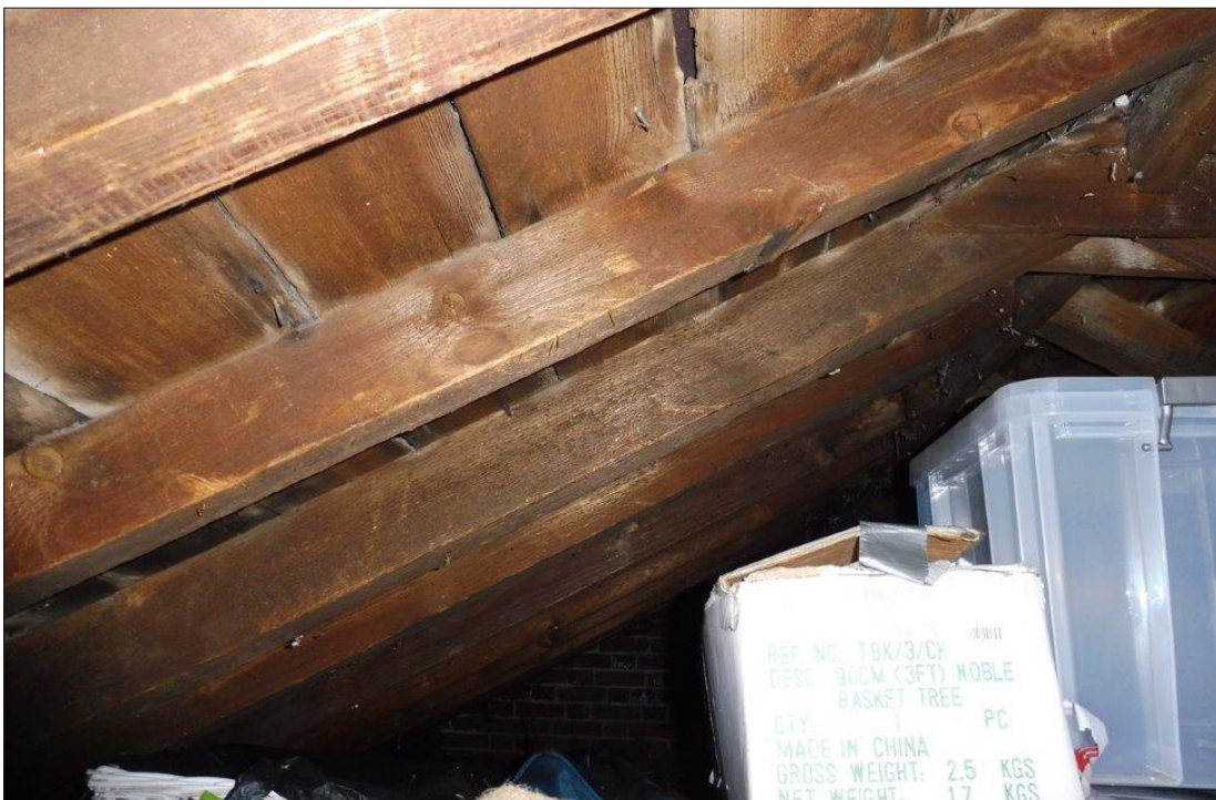
PHOTOGRAPH 2: Loft Void within Building B1a
