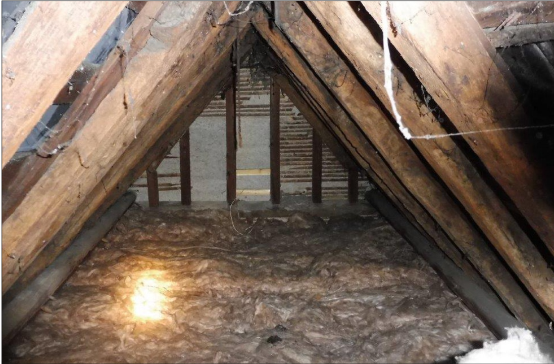
PHOTOGRAPH 3: Loft Void within Building B1b
