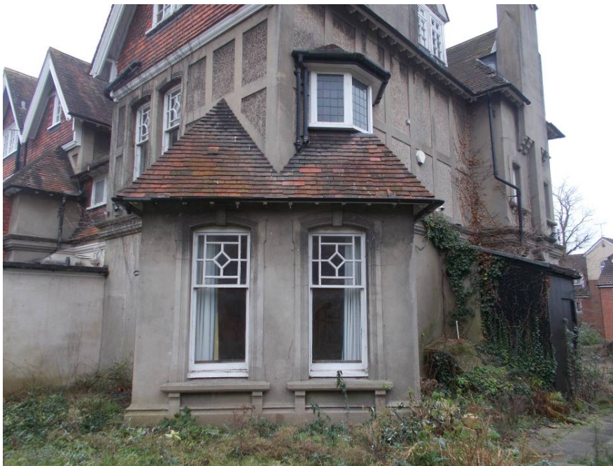
Rear asymmetrical form with vertical sliding sash windows
