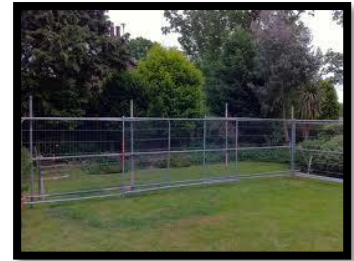
TREE PROTECTION BY HERAS PANELS OR MARINE BOARD BOXING
