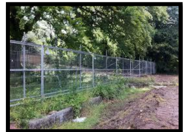
TREE PROTECTION BY HERAS PANELS OR MARINE BOARD BOXING
