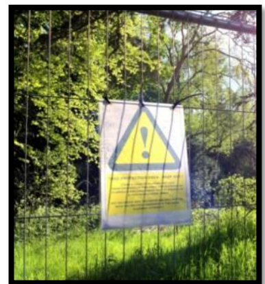
ALL WEATHER SIGNAGE (SHOWN IN APPENDIX D) DISPLAYED ON HERAS PANELS
