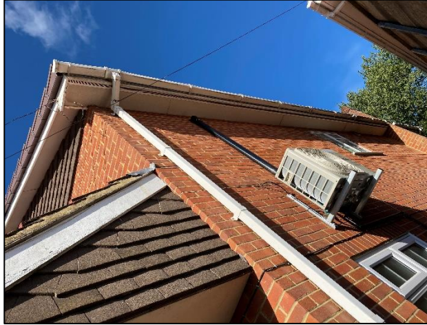
Photo 2: The eastern elevation of B1.
