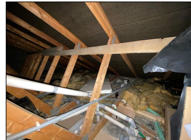
Photo 12: Inaccessible crawl space in Loft 1.
