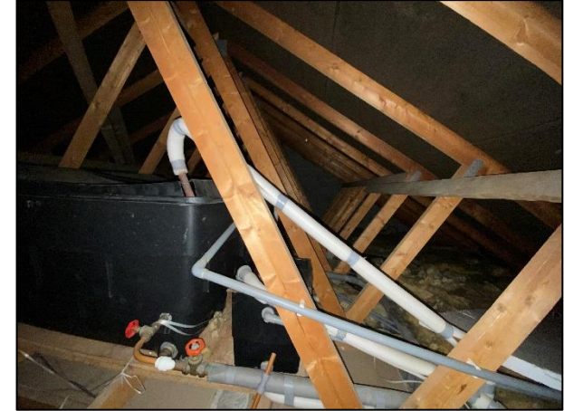
Photo 9: Inaccessible area of the loft.
