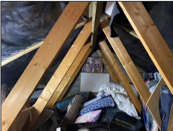
Photo 10: Loft space lined with plastic sheeting.
