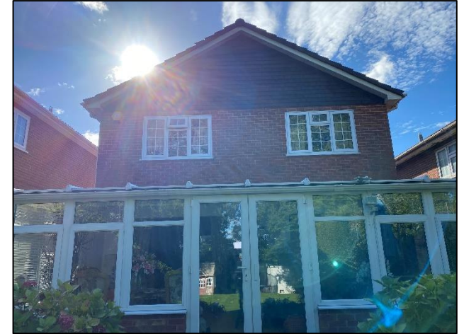
Photo 3: The northern elevation of B1.
