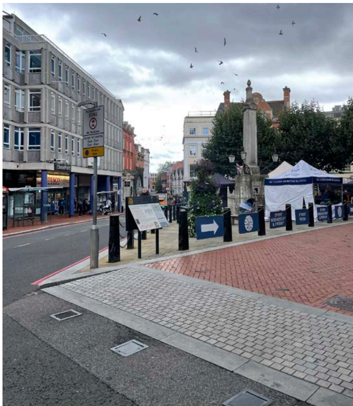
View looking south down Market Place with 6 – 8 Market Place to the left.
