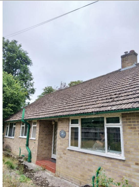
Photograph 8 – West aspect of B1.
