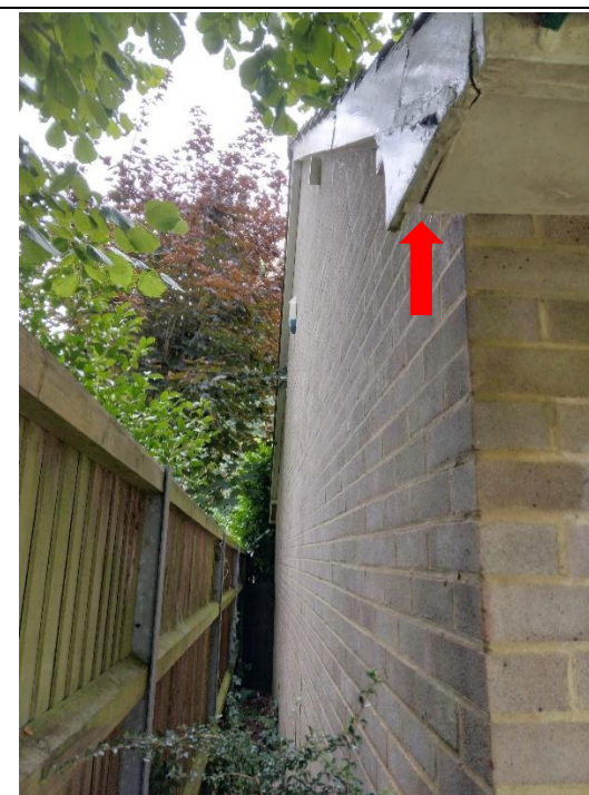
Photograph 13 – north gable end of B2.
