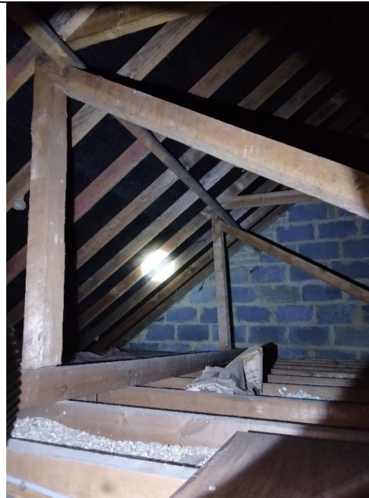
Photograph 14 – Internal view of the loft space within B1.
