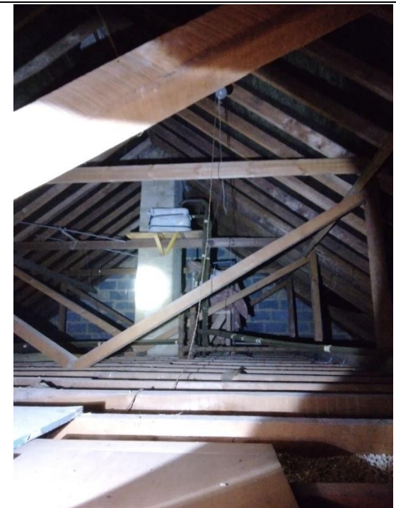
Photograph 15 – Internal view of the loft space within B1.
