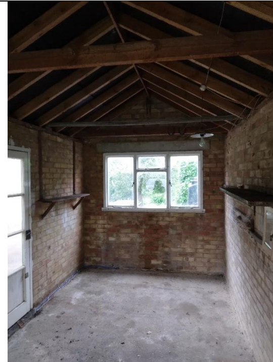
Photograph 18 – Internal conditions of B2.
