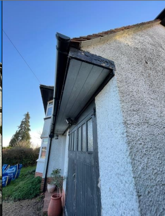
Photograph 6: Eastern aspect soffits above garage in good condition.
