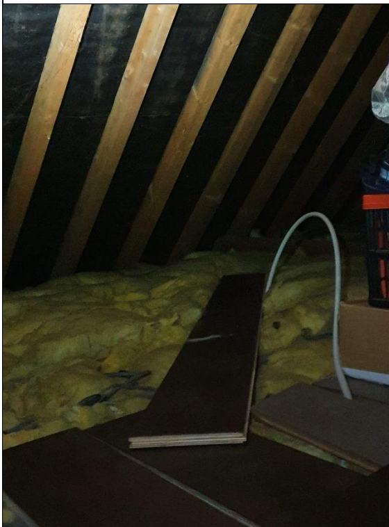
Photograph 11: Loft space with fibreglass insulation.
