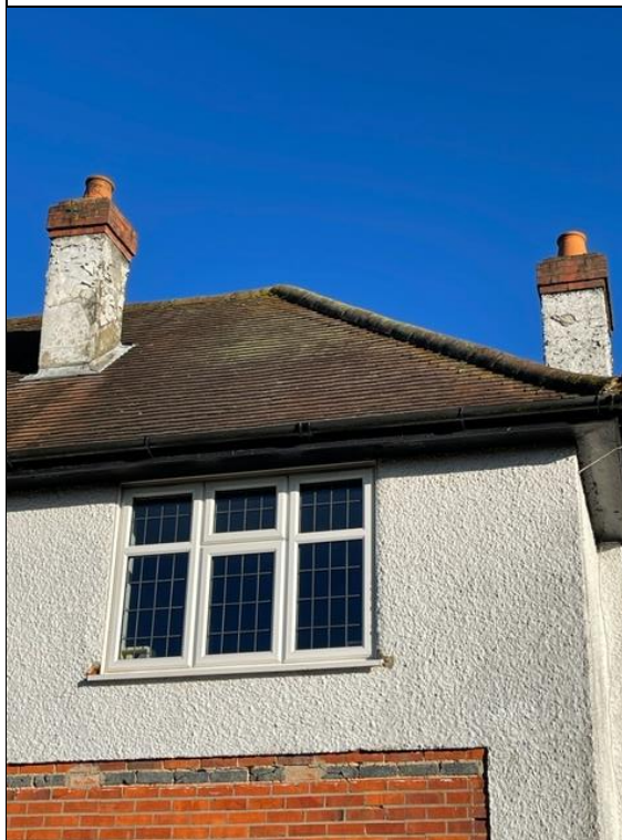
Photograph 3: Western aspect with clay roof tiles in good condition.
