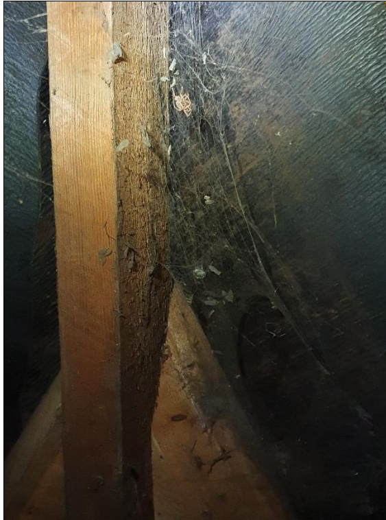
Photograph 13: Lining in good condition no tears or rips and no visible gaps.
