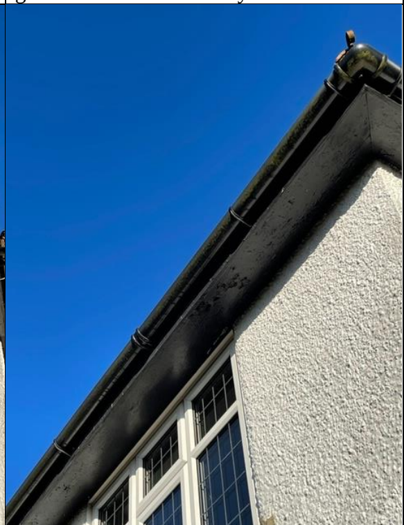
Photograph 4: Wooden soffits, in good condition no shrinking.
