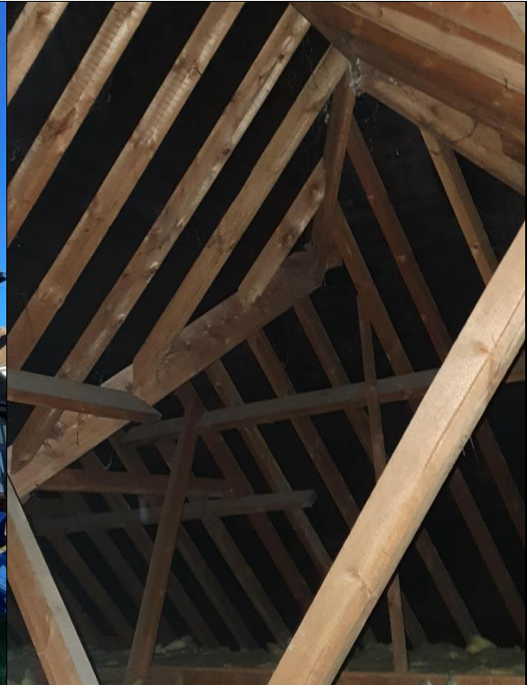
Photograph 10: Black bitumen lined loft space in good condition.
