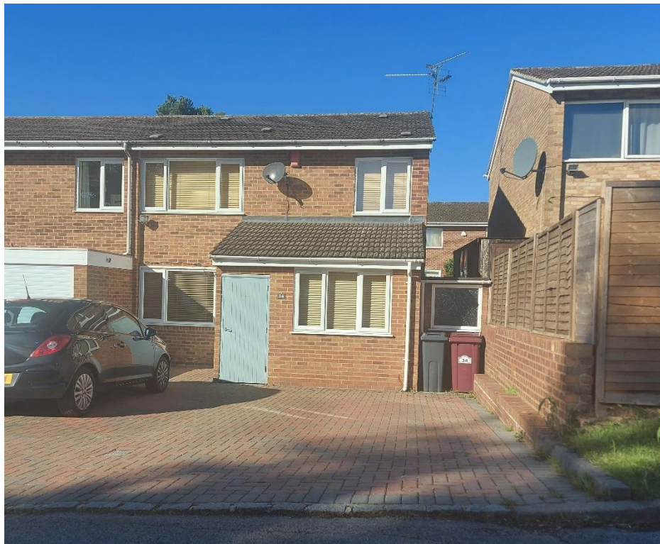
1 Photograph of the front elevation of 34 Harlech Avenue, taken at site visit on 21.10.2021
