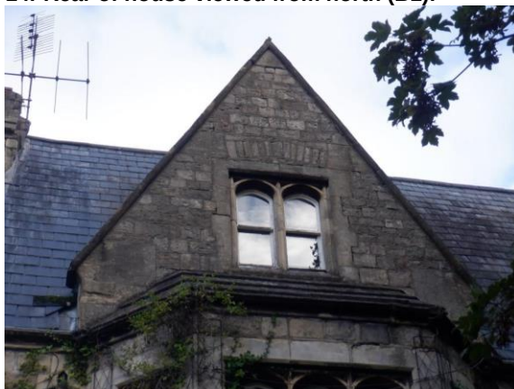
16. Additional gable on southern side of house (southern elevation).
