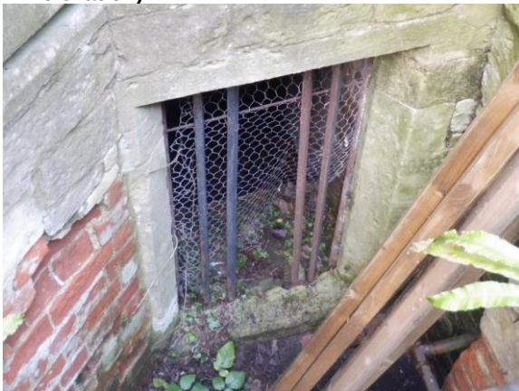
23. Basement window (eastern elevation).
