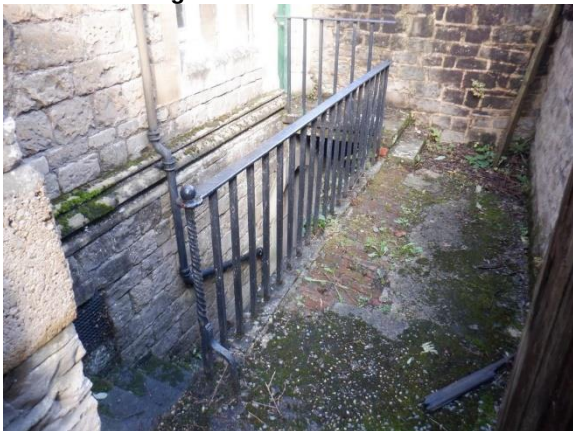
35. Entrance to basement.
