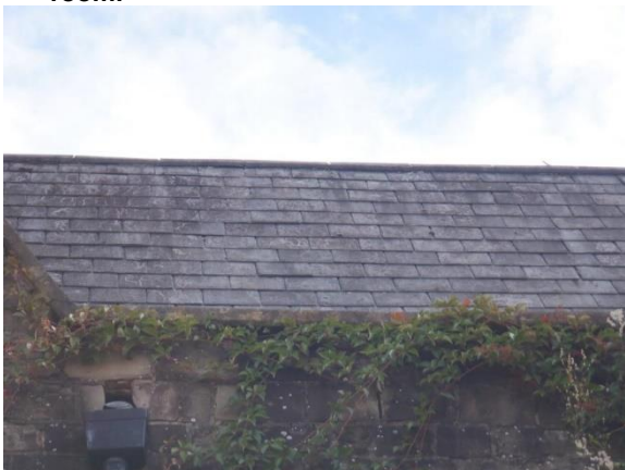
17. Slate roof tiles flat and intact (western elevation).
