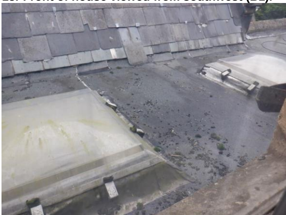
15. Central bituminous flat roof viewed from attic room.
