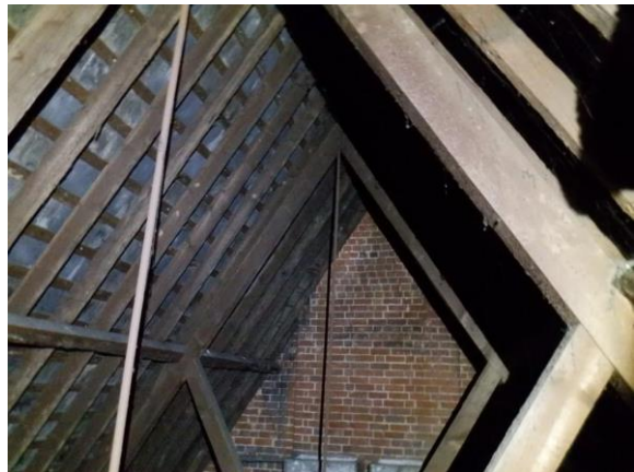
24. Northern side of roof void.
