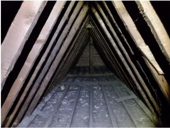
31. Southern section of roof void.
