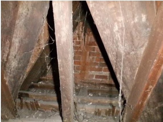
33. Additional gable end above attic room.
