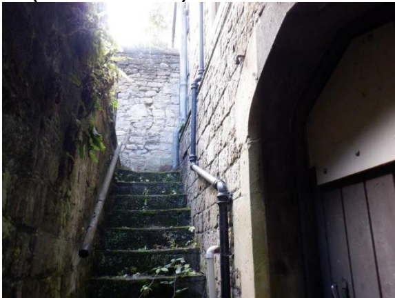
21. Steps leading down to basement (eastern elevation).
