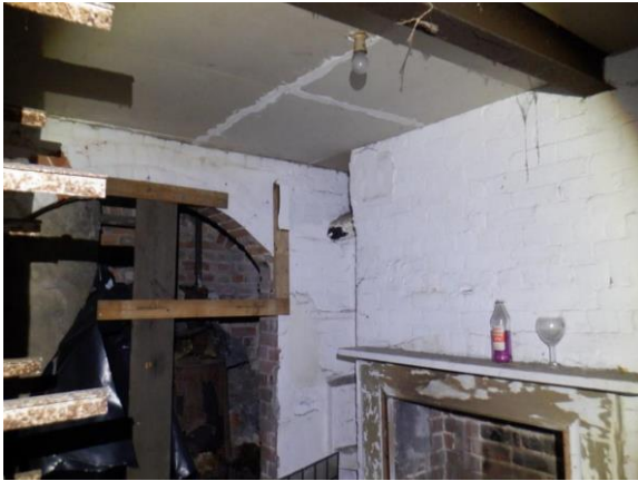
37. Old boiler and disused fireplace.
