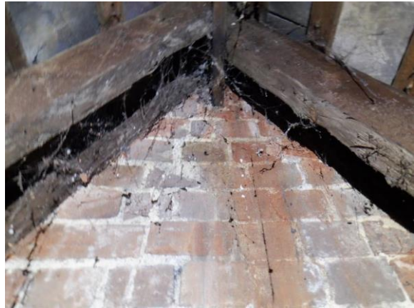
32. Heavily cobwebbed gable end.
