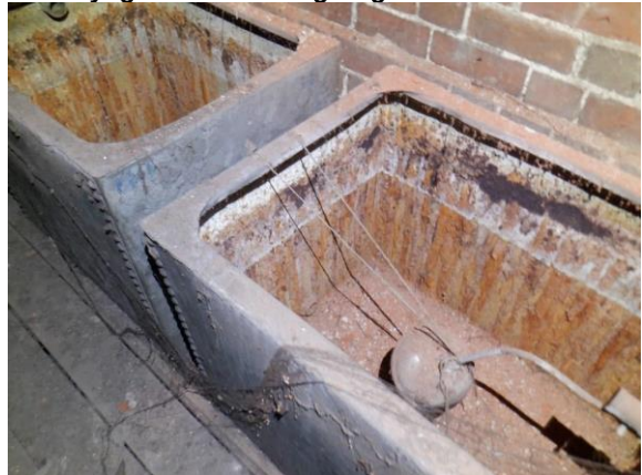
28. Two empty water tanks at north-eastern gable end.
