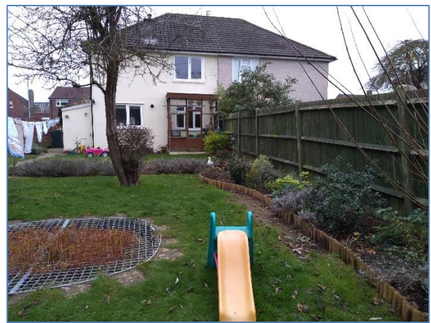
2. Rear and side of 22 Brayford Road. Photo provided by the agent on 28/11/2020.
