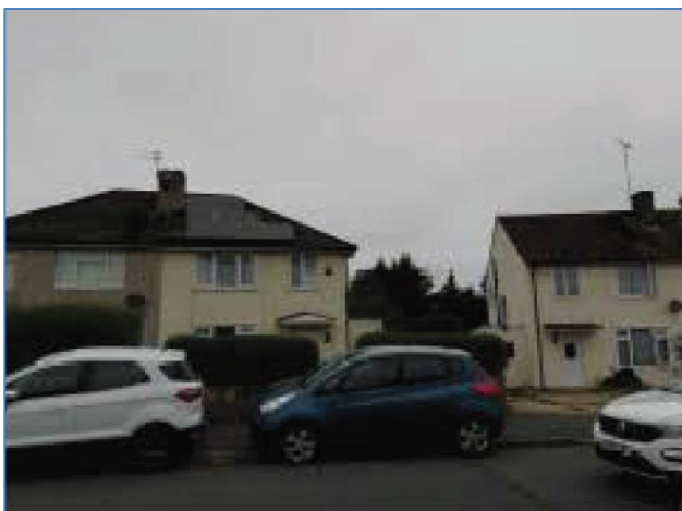
1. Front of 22 Brayford Road. Photo provided by the agent on 21/11/2020.
