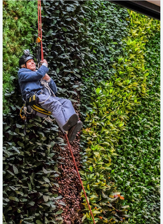
David Attenborough Building, installed in 2016
