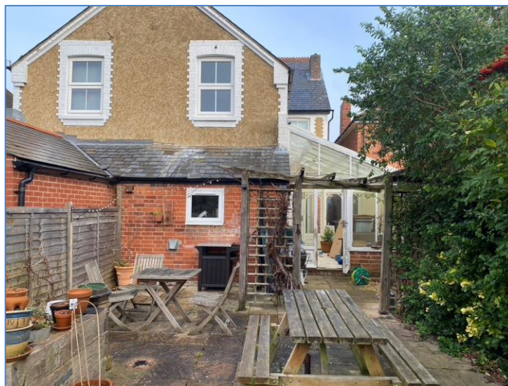
1. Rear of 68 Recreation Road. Photo provided by the agent on 23/11/2020.
