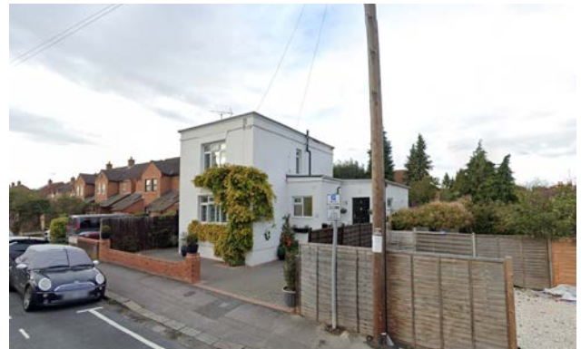
Figure 1-7. View D - 4 Montague Street
