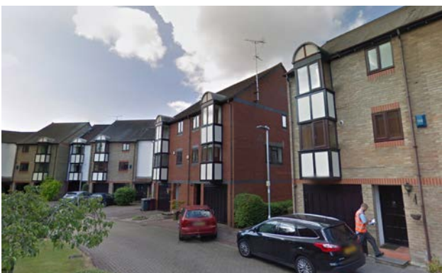
Figure 1-11. View G - Heron Island Flats
