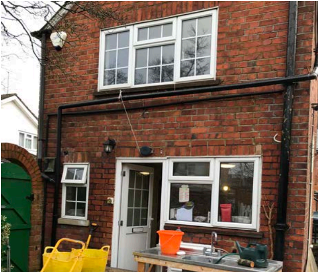
Figure 1-18. G - View toward western elevation
