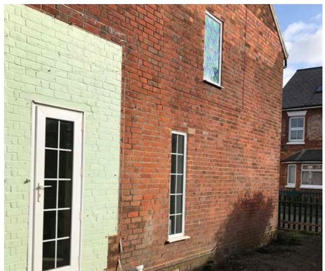
Figure 1-17. F - Lower southern elevation
