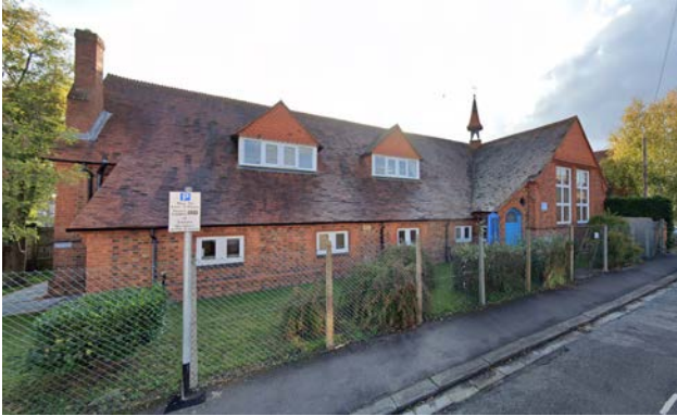
Figure 1-4. View A - Caversham Hall
