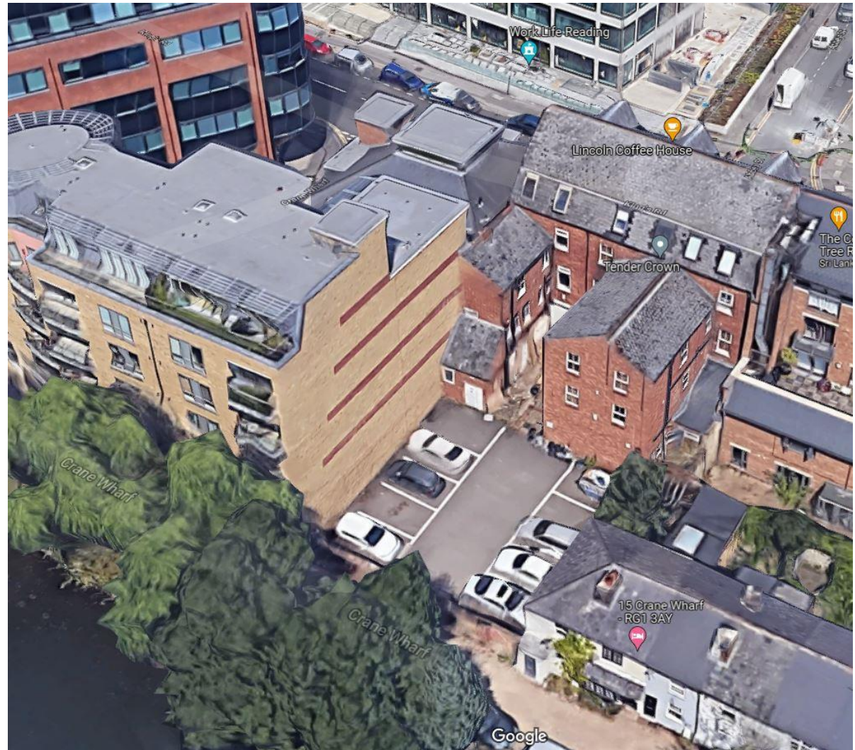
Figure 2 - 3d Arial View of the Site
